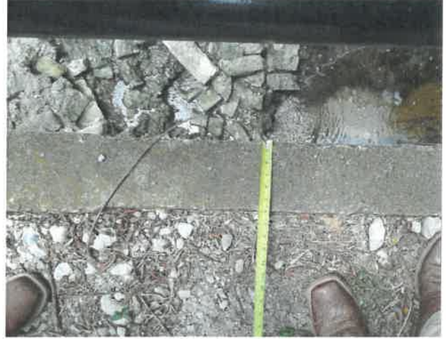
Headwall thickness varies from 6" to 8"
