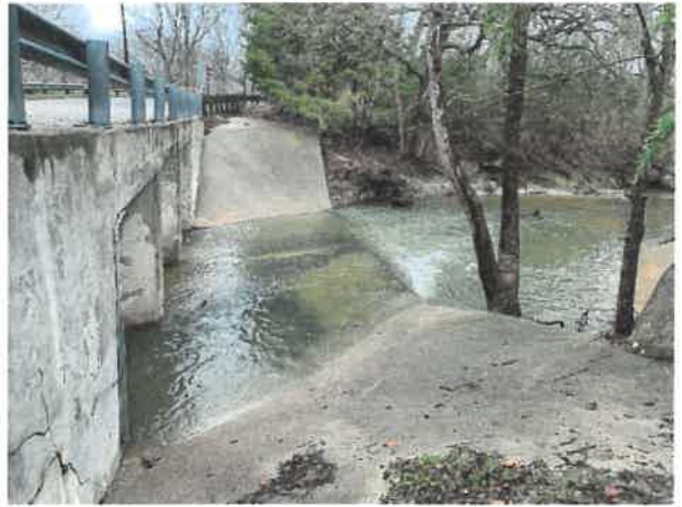
Downstream Headwall
