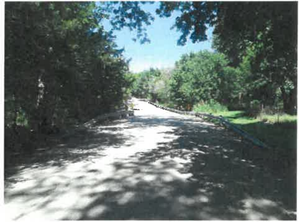
Approach - Looking West
