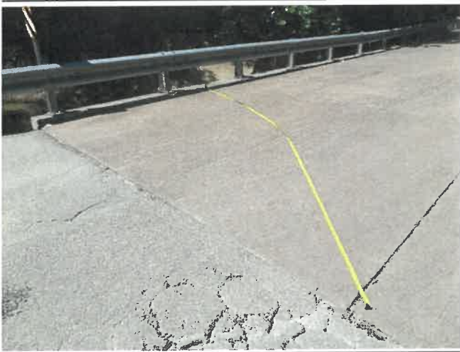
1/8" diagonal crack
