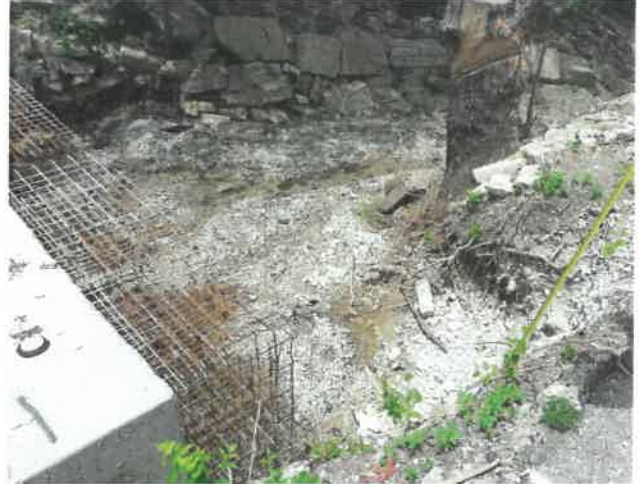
6' drop off 1' off the road (currently under construction)
