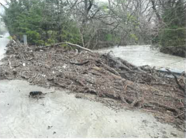
At Snider Lane Culvert – During A Storm Event
