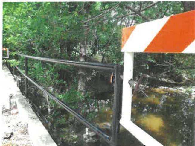
Railing/gate connection in good condition
