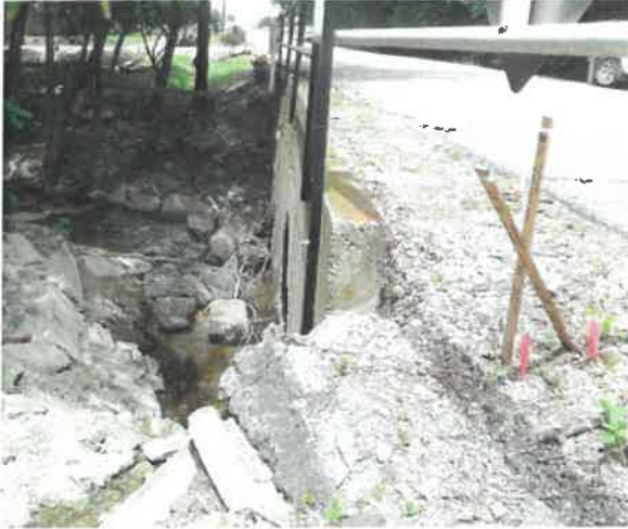
Typical - no deficiencies noted.
