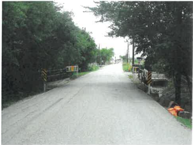
Approach - Looking South
