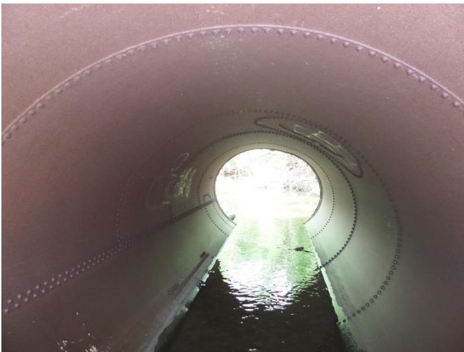
Typical – no deficiencies noted
