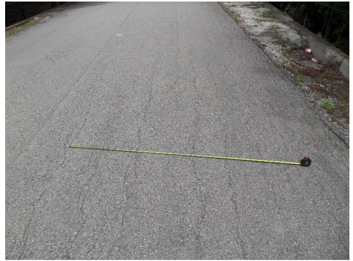
Right Lane substantial longitudinal cracking.
