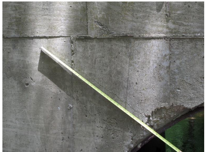
16" x 5" x 1.5" spall and 36" x 0.05" crack near culvert 1
