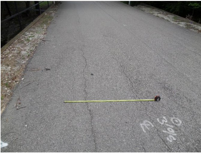
Left lane with Marginal longitudinal cracking (Typ.).
