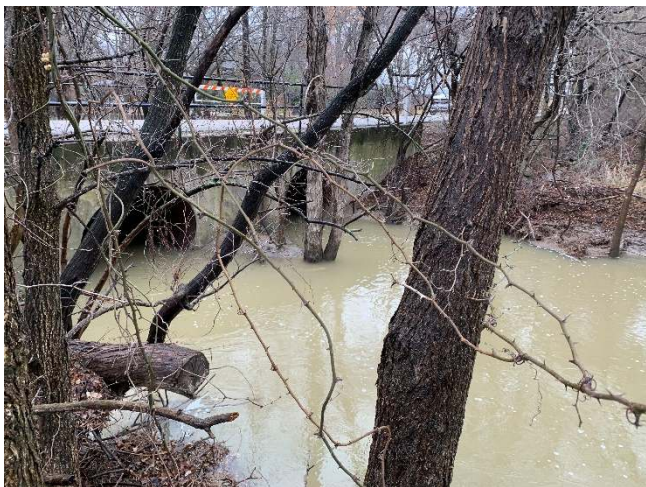
Downstream – During A Storm Event
