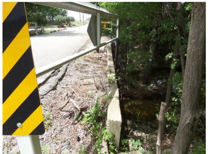
Headwall 2 out of plumb
