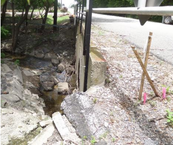
Typical - no deficiencies noted.
