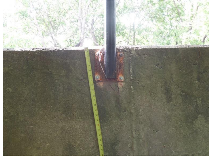
3" x .05" crack at first railing support connection to headwall 2
