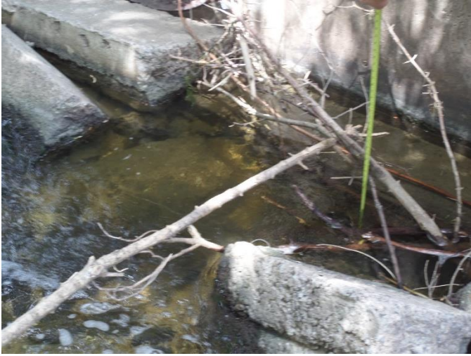
Undermining of headwall 1 at midspan
