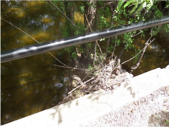
Evidence of flooding
