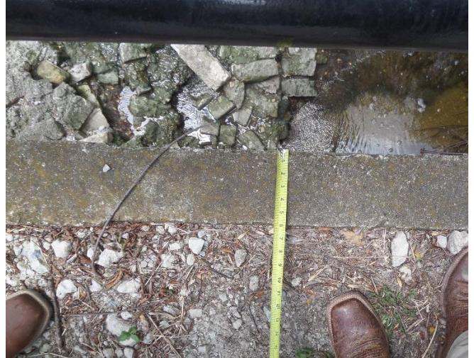
Headwall thickness varies from 6" to 8"
