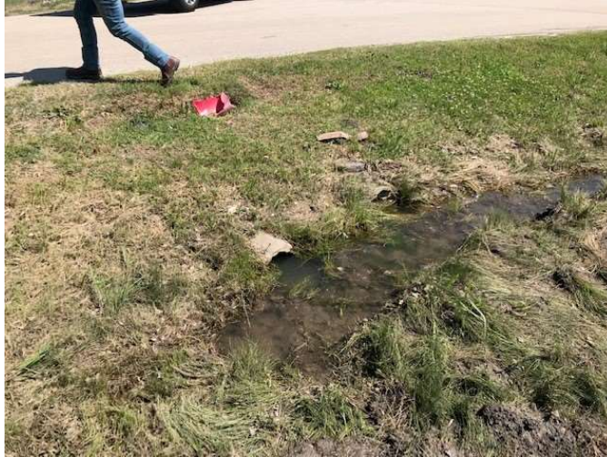
Image 1: Downstream Face of Mandarin Cove Culvert
