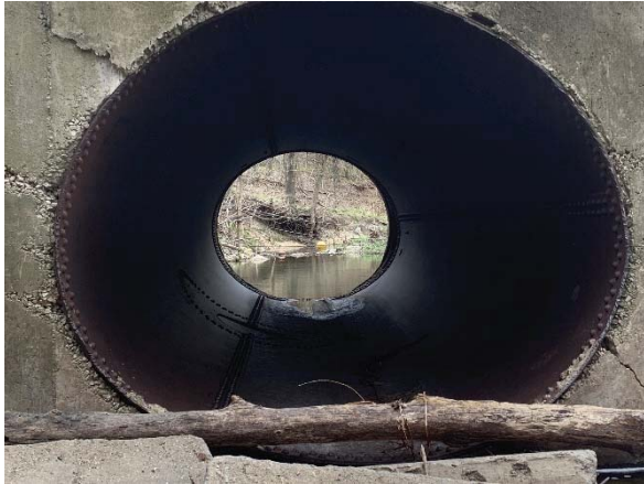
Typical – no deficiencies noted
