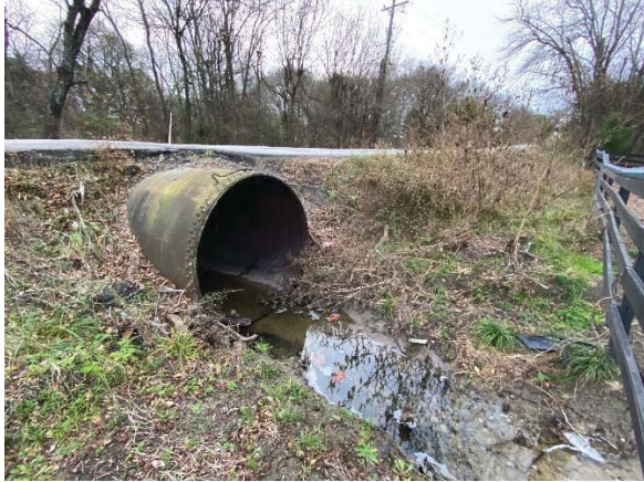
Bank erosion & scour.
