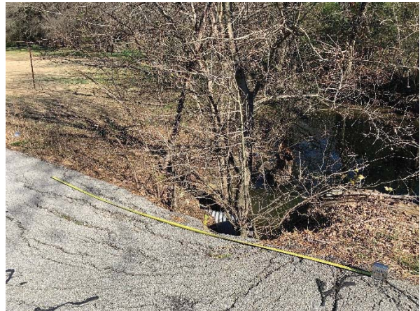
8-1/2' of erosion on NE corner of pipe
