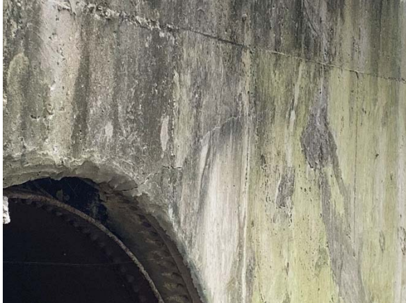
Horizontal crack
