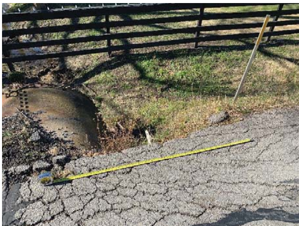
4' of erosion on NW corner of pipe
