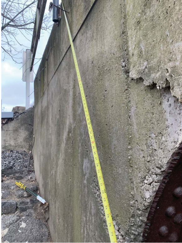
Spall, Crack – 6.5' x 0.035" N of Culvert 1
