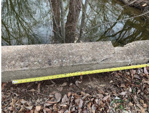
Crack, Spall – 10" x 5" x 2.5"
