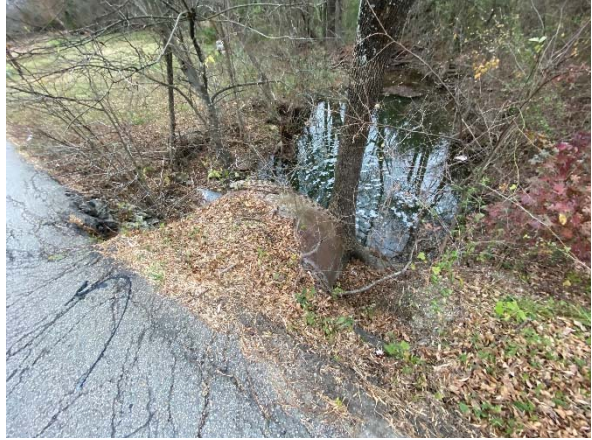
Bank erosion & scour.
