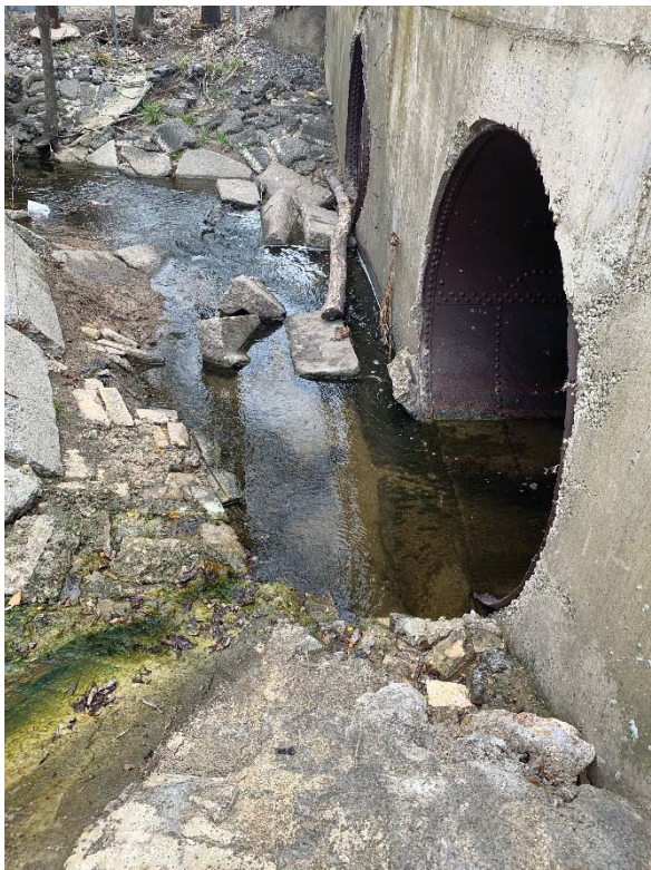
Undermining at headwall 2
