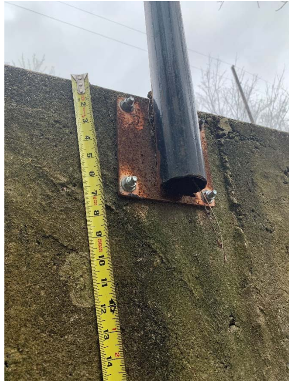
Crack at SE railing support – 10" x 0.08"
