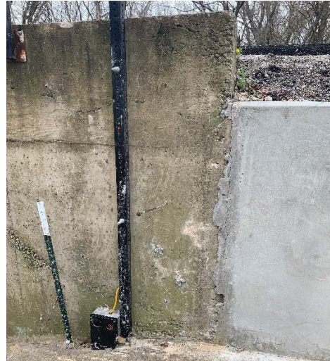
Crack at joint of headwall 2 and new wingwall
