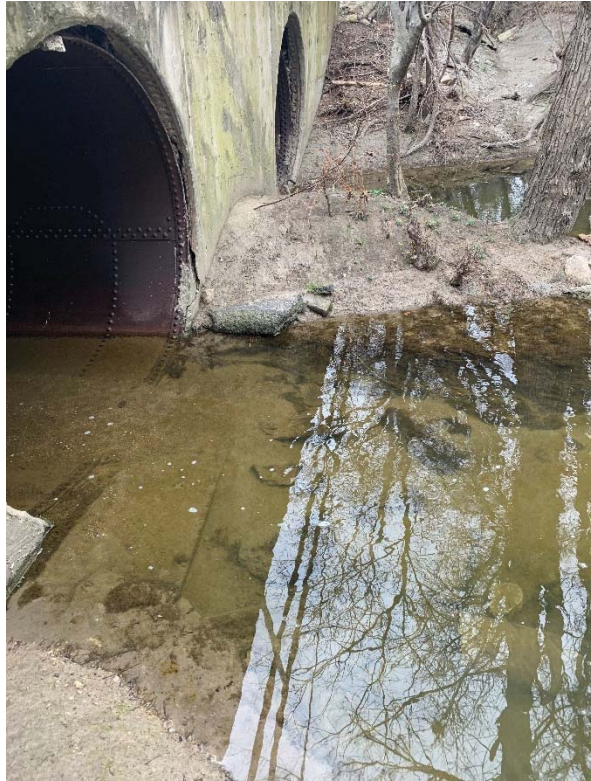
Undermining at headwall 1
