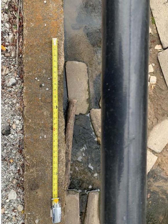
Midspan Spall – 10" x 4" x 1"
