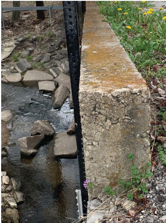
Typical – No deficiencies noted
