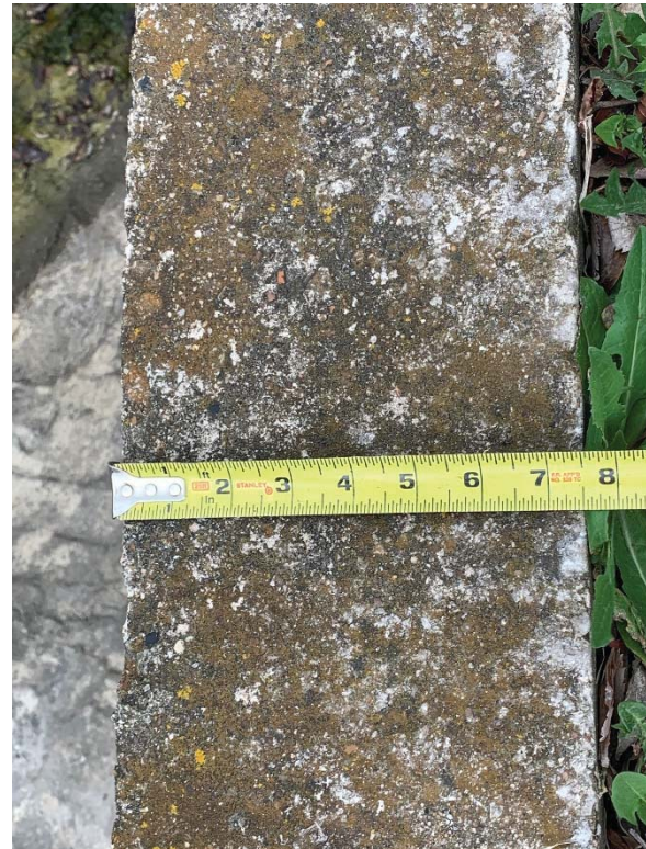
Headwall thickness varies from 6" to 8"
