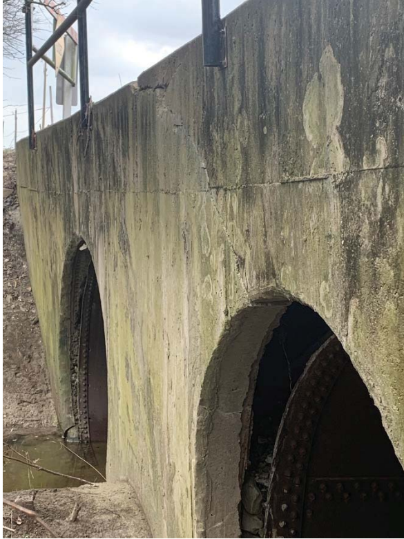
Full Depth Crack
