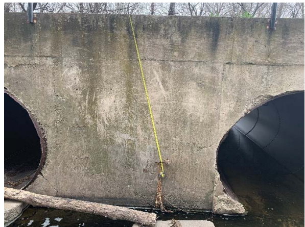
Full depth crack down headwall – 7.5' x 0.030"
