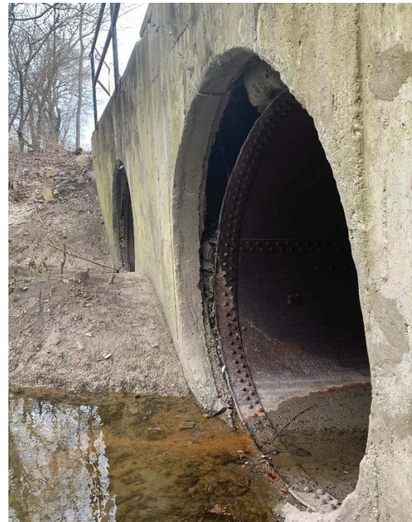
Loss of backfill at outlet headwall above pipe
