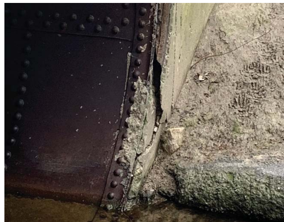
Spall – likely a result of construction
