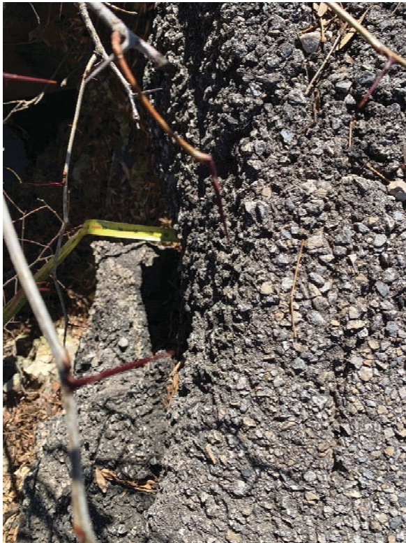
Road undermined 4" on NE corner.
