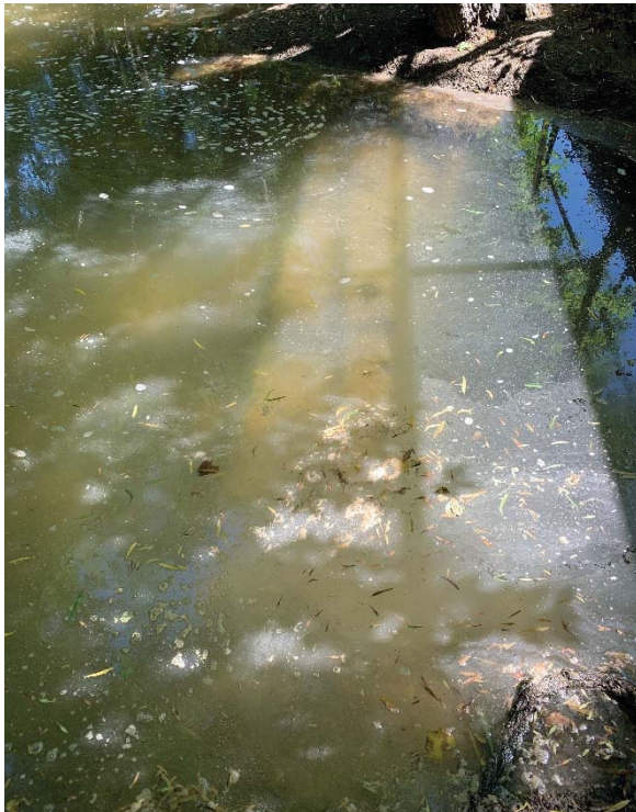
Approx. 1.5' scour exposing encased utility
