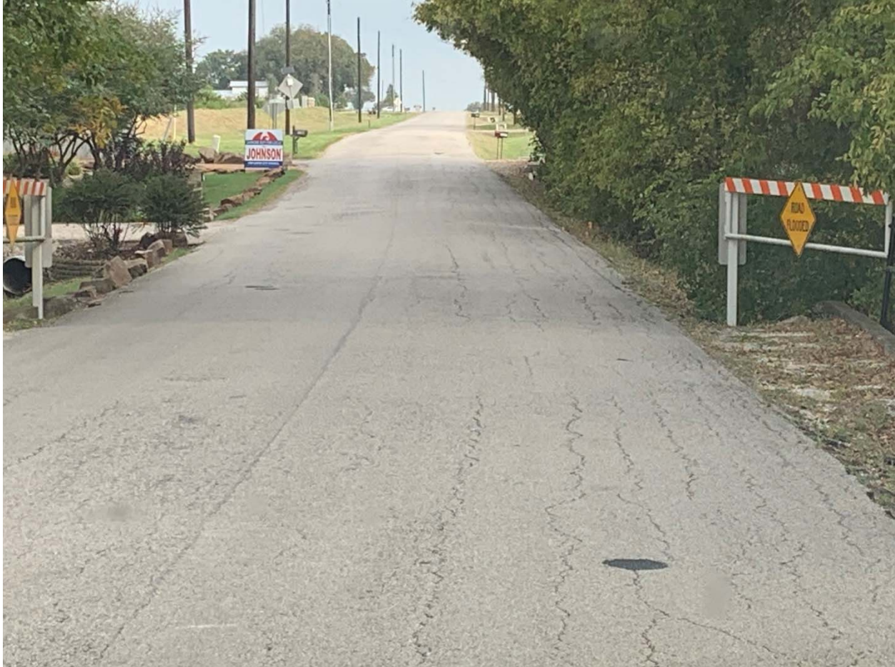
NB Lane - substantial longitudinal cracking
