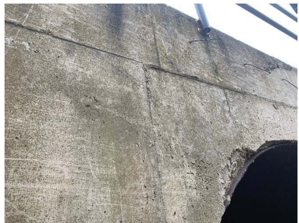
Spall – 16.25" x 5" x 1.5", Crack – 3' x 0.05"
