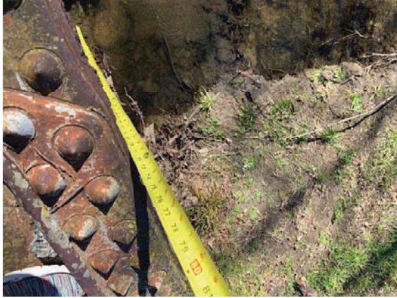
12: Culvert Height – West Side
