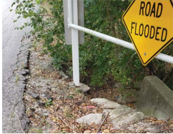
Pavement edge failure – all four corners (TYP)
