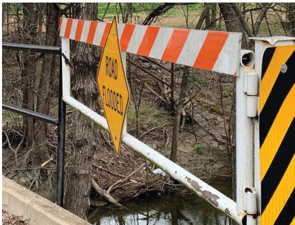
Railing and gate connection in good condition
