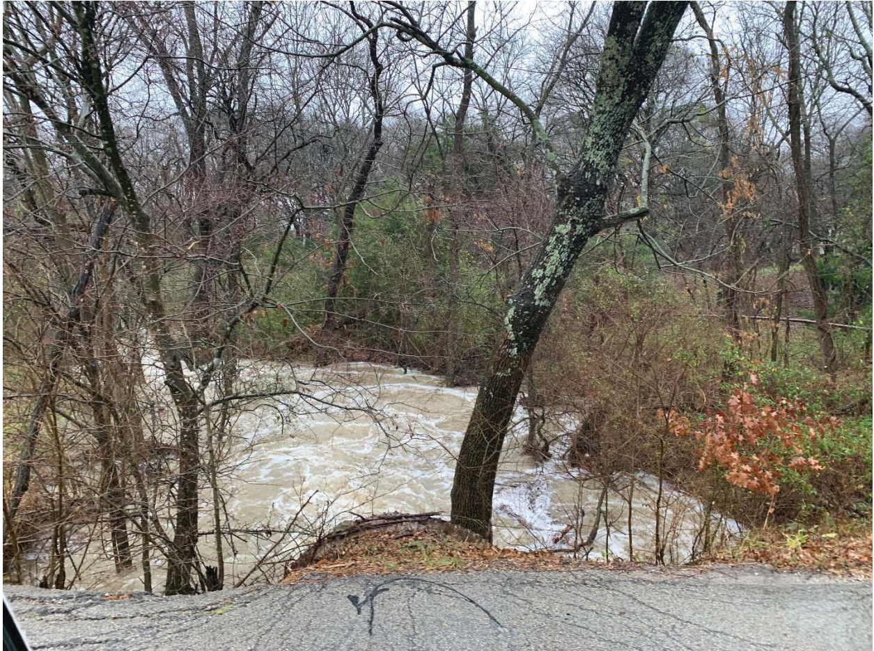
Disruption of water flow due to tree and debris
