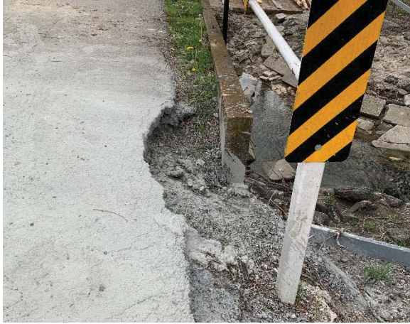
Substantial pavement failure (14")
