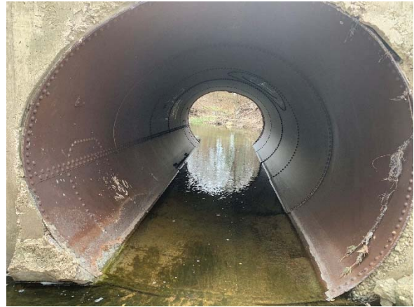
Sediment build-up along bottom
