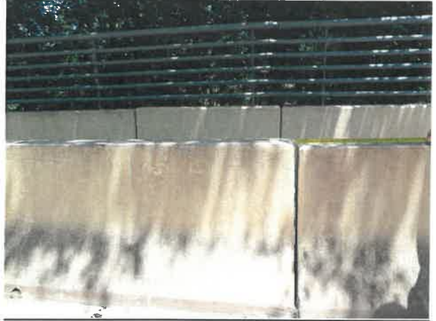
Approach slab 1 rotated up 1/2" at end bridge southeast corner
