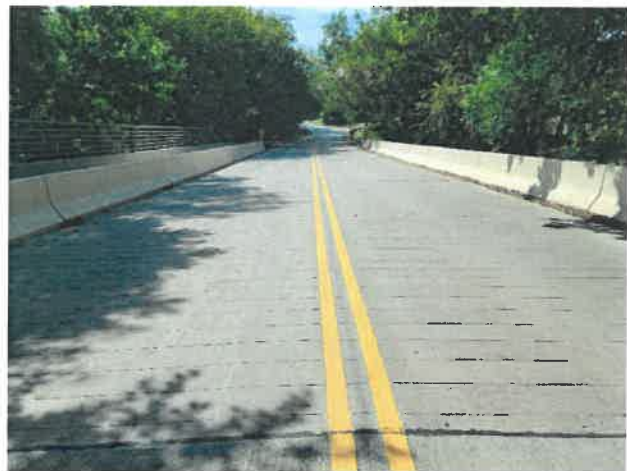
N. Approach - Looking South
