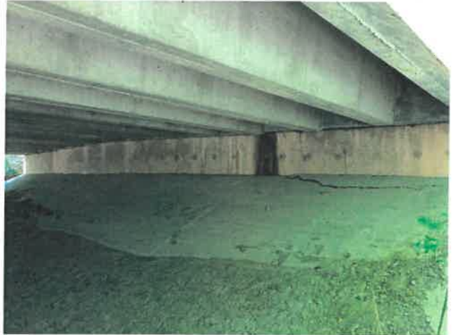
25: Abutment 2 – Looking Northwest
