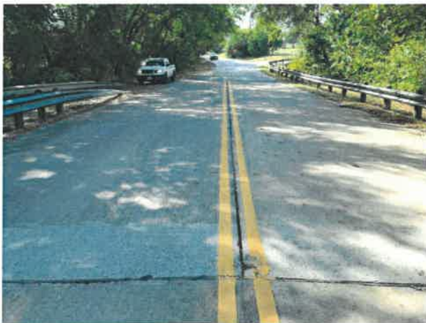
Joint - S. Approach Slab
