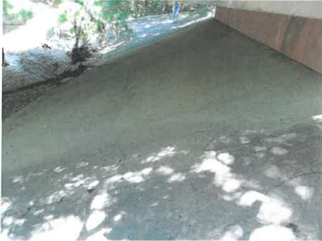
Typical – no deficiencies noted
