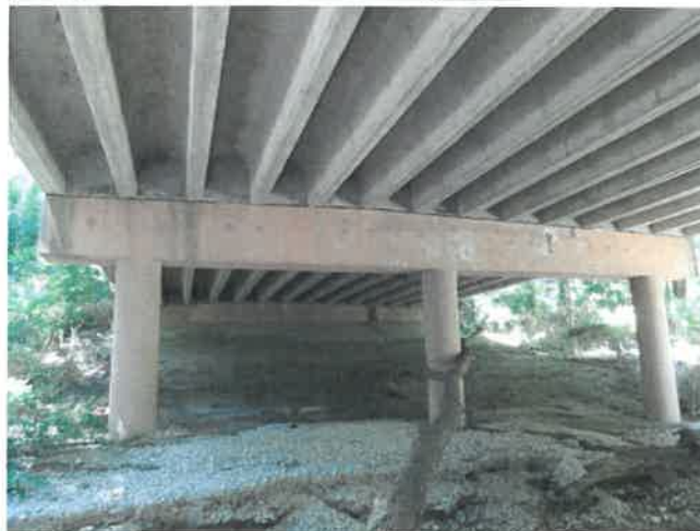
19: Span 2 – Under View – Looking North
