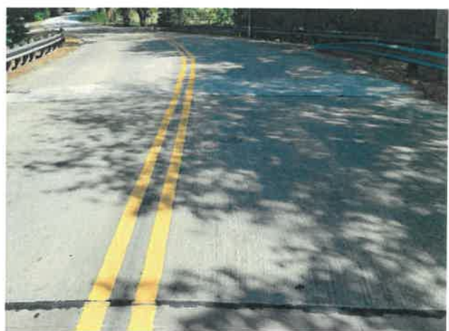
Joint - N. Approach Slab
