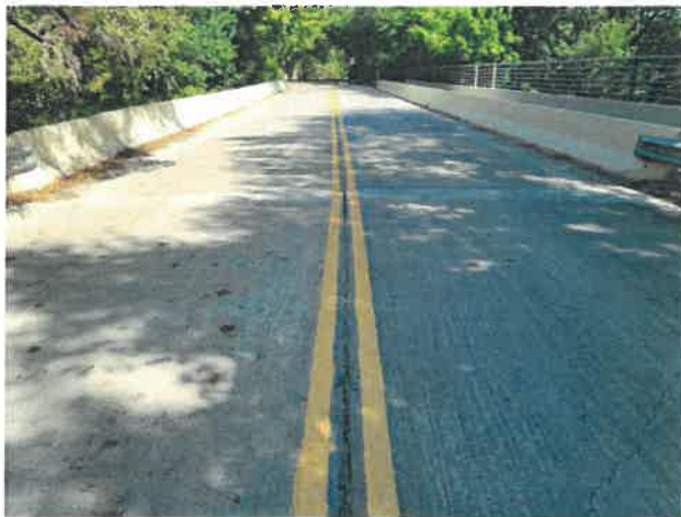
S. Approach - Looking North
