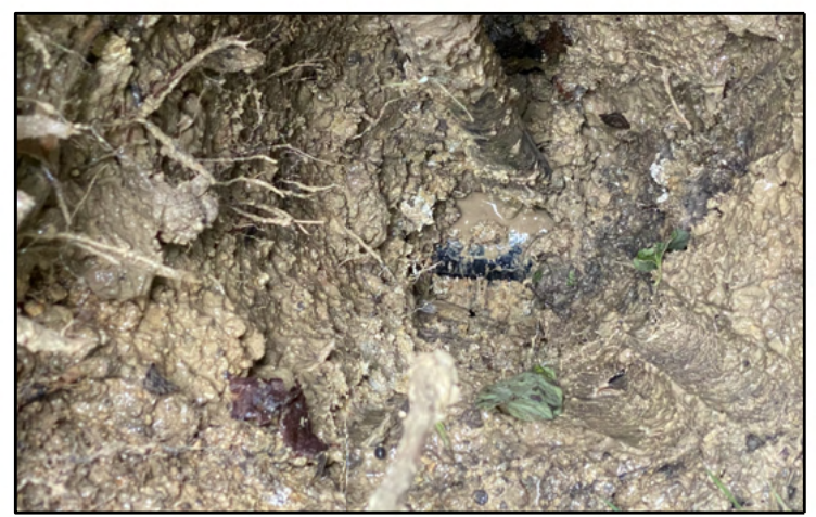
TEST HOLE PHOTO OF UTILITY
