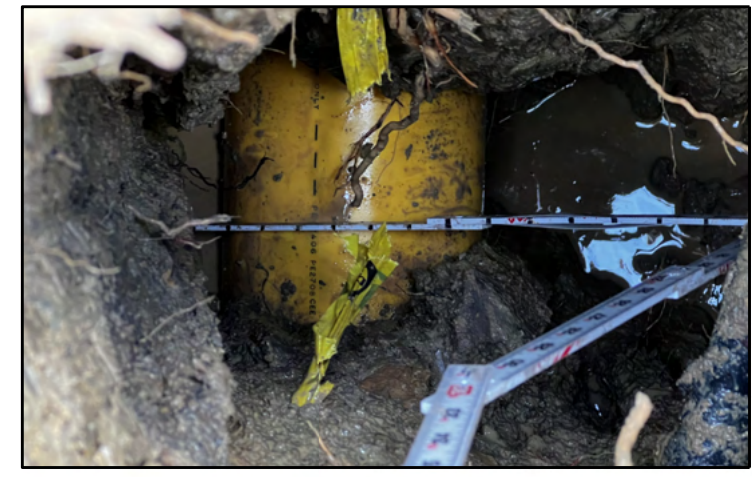
TEST HOLE PHOTO OF UTILITY
