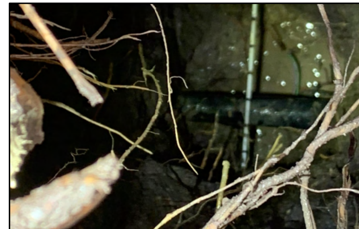
TEST HOLE PHOTO OF UTILITY
