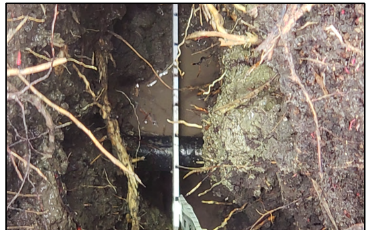
TEST HOLE PHOTO OF UTILITY
