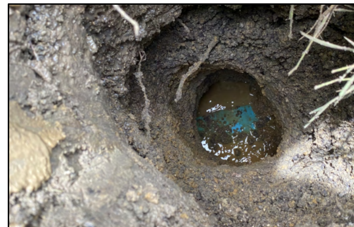
TEST HOLE PHOTO OF UTILITY
