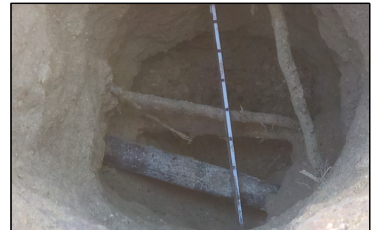
TEST HOLE PHOTO OF UTILITY
