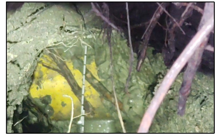
TEST HOLE PHOTO OF UTILITY
