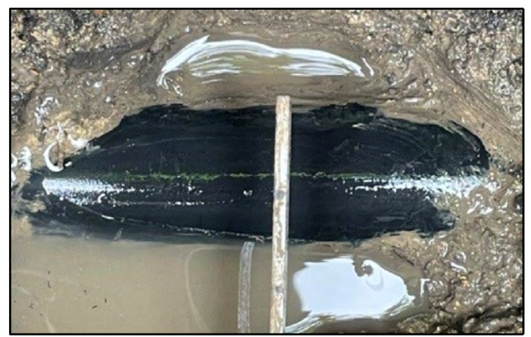
TEST HOLE PHOTO OF UTILITY
