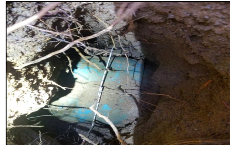
TEST HOLE PHOTO OF UTILITY
