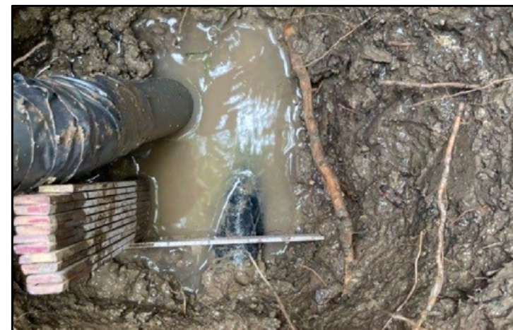
TEST HOLE PHOTO OF UTILITY
