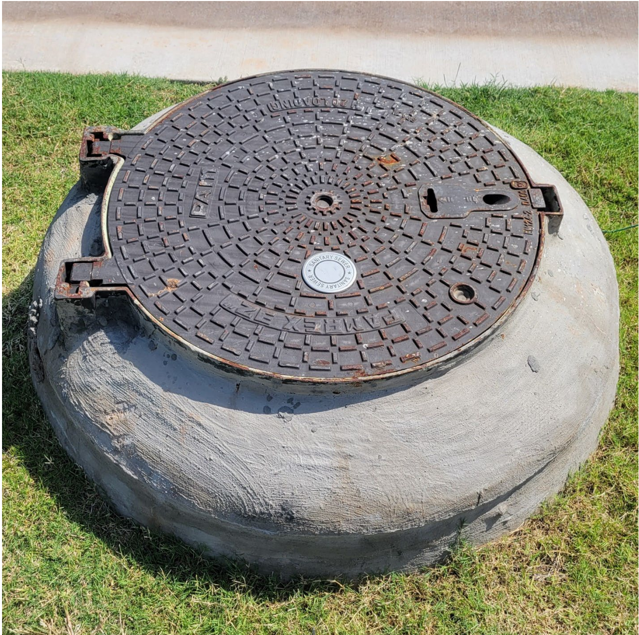
(Image: Manhole at Lucas Retail Addition)
