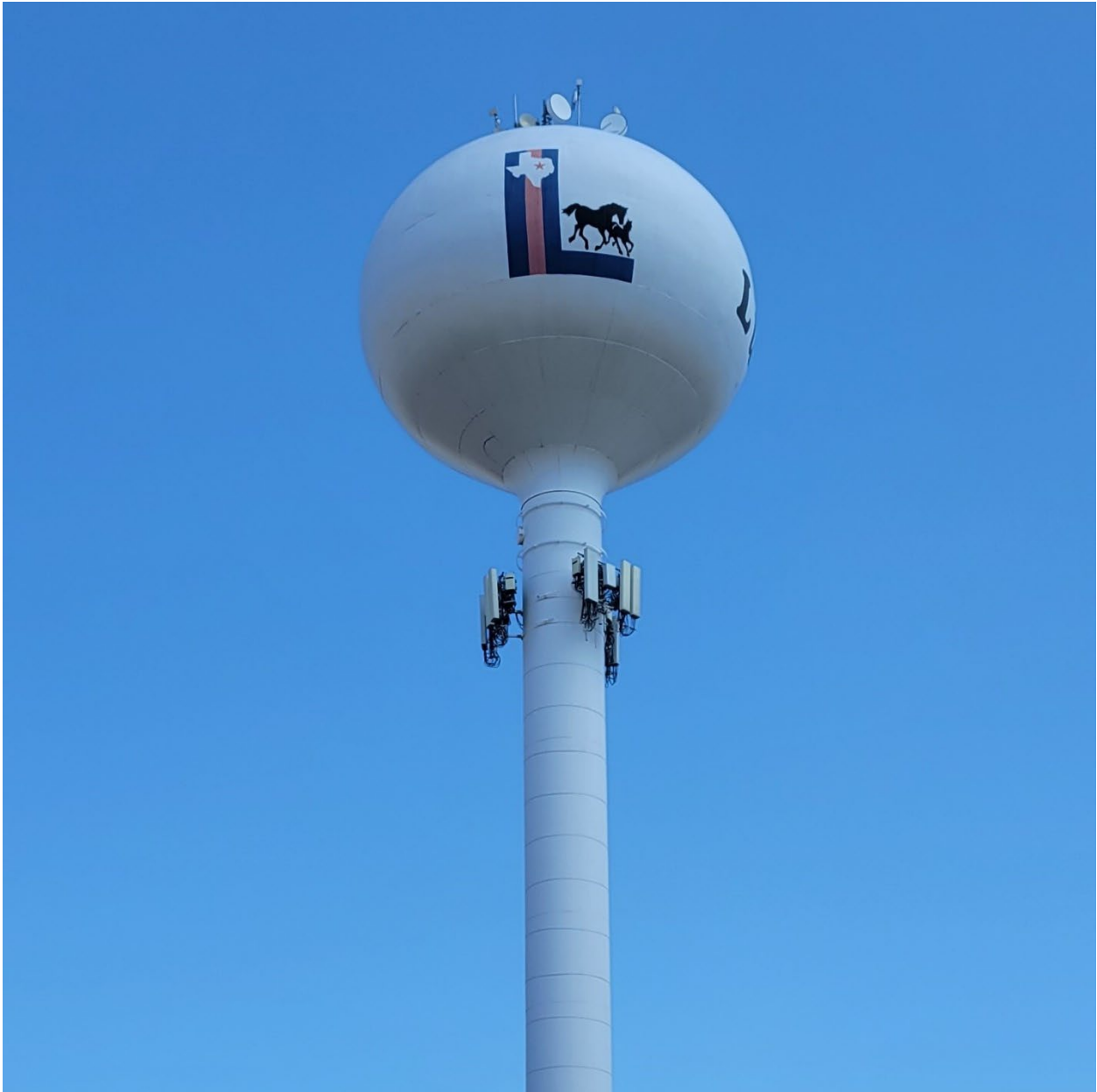
(Image: Winningkoff Water Tower)
