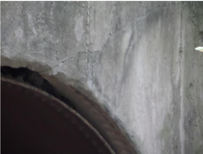
5' Horizontal crack near culvert 1
