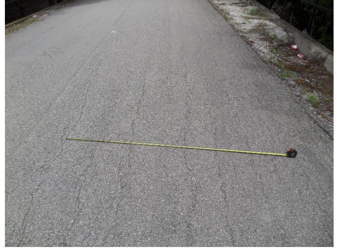
Right Lane substantial longitudinal cracking.
