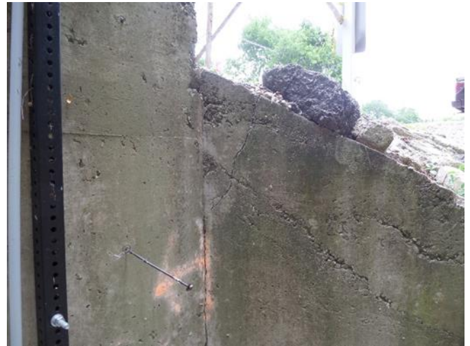
19" x 1/8" crack at wingwall 1
