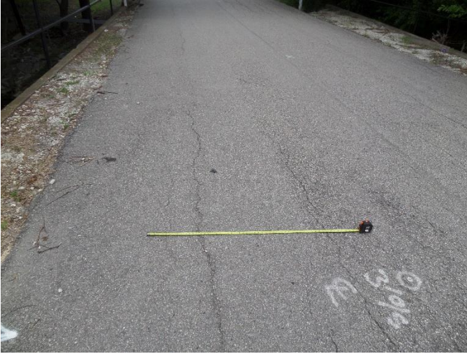
Left lane with Marginal longitudinal cracking (Typ.).
