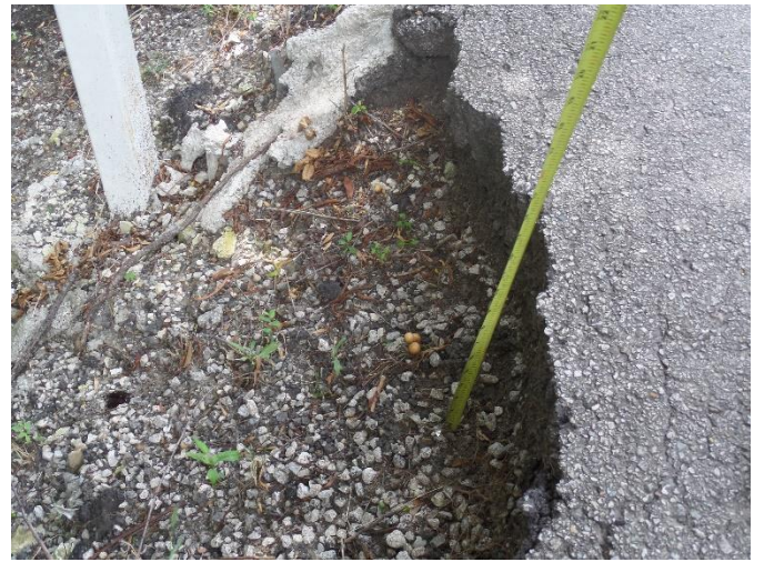
Substantial pavement failure (12")
