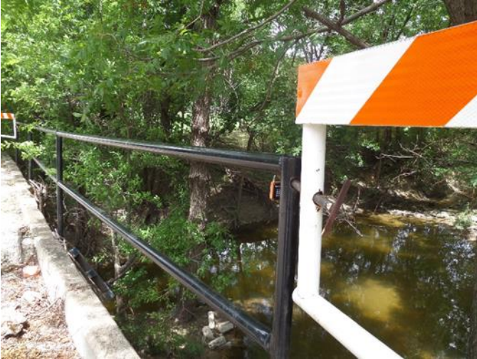
Railing/gate connection in good condition
