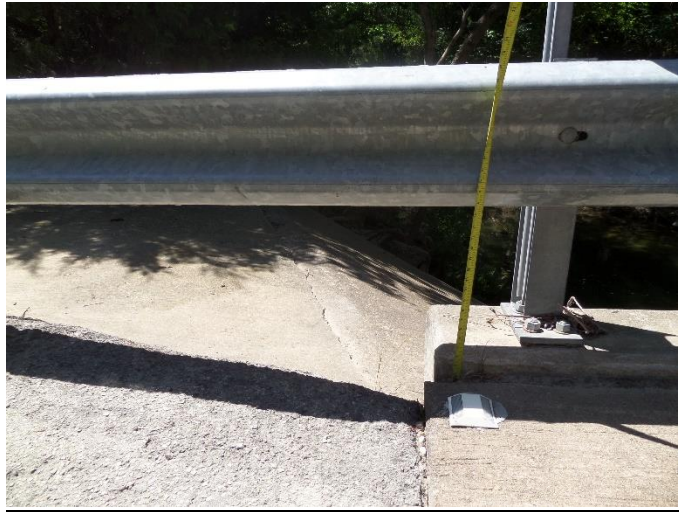
2-1/2" settlement of approach slab 2
