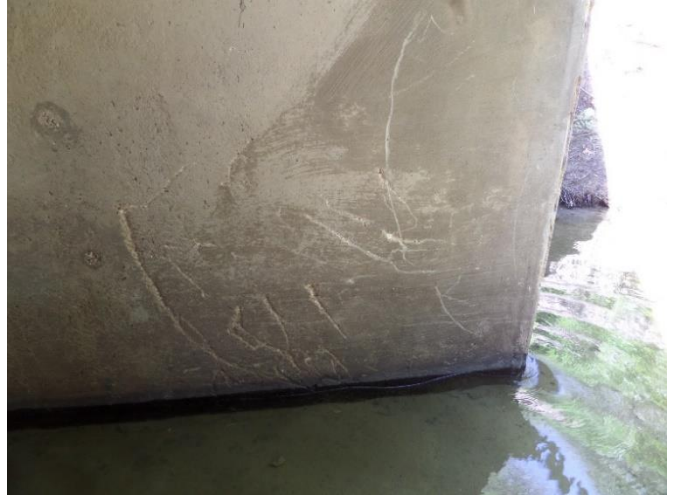
Scaring and gouging from debris at northwest corner (Typ.)
