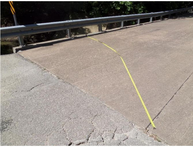
1/8" diagonal crack
