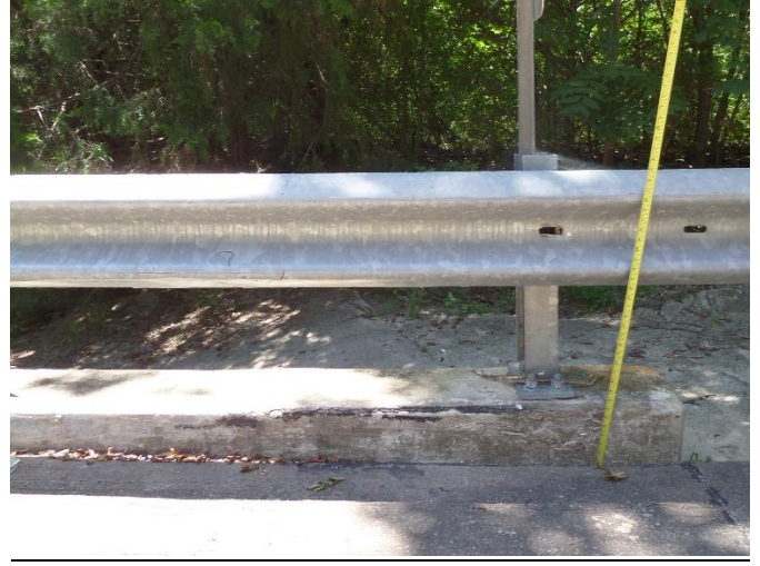
6" settlement of approach slab in southwest corner
