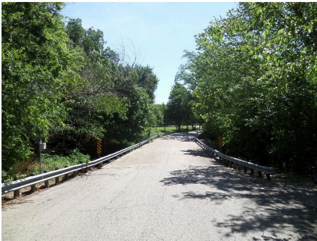
Approach- Looking East
