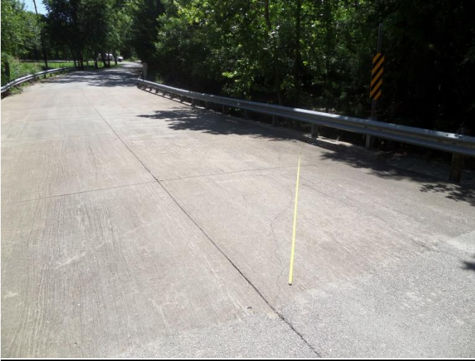
Diagonal crack at southwest portion of approach
