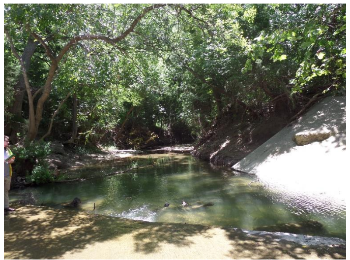
Moderate bank erosion looking downstream
