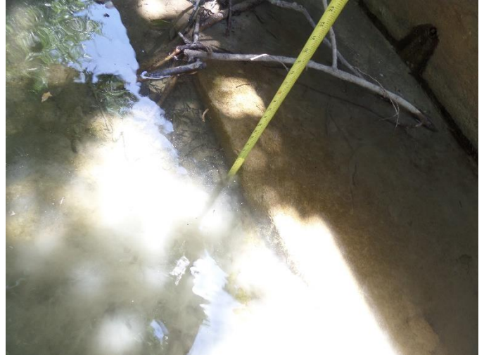
5" scour at bottom slab toe, northeast corner
