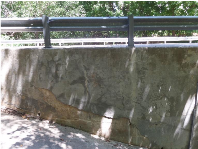
75% delaminated on southwest face abutment 1
