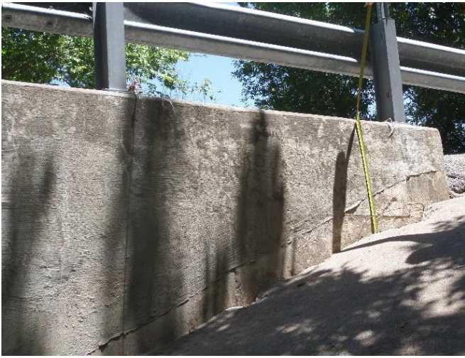
Concrete riprap settled 9"
