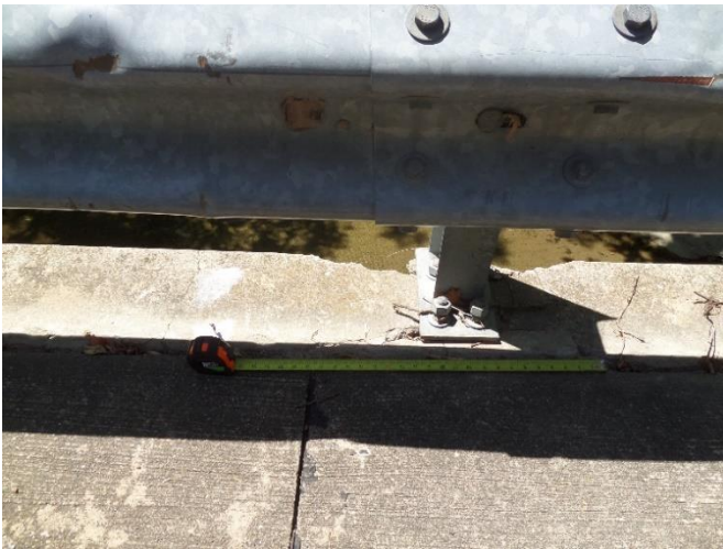
7" x 24" x 3" spall at the second post of span 2
