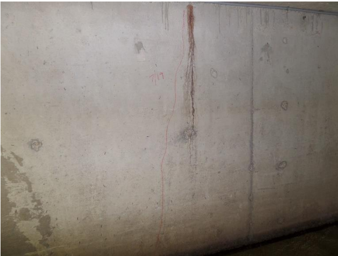
0.010" crack full height at 10' with efflorescence
