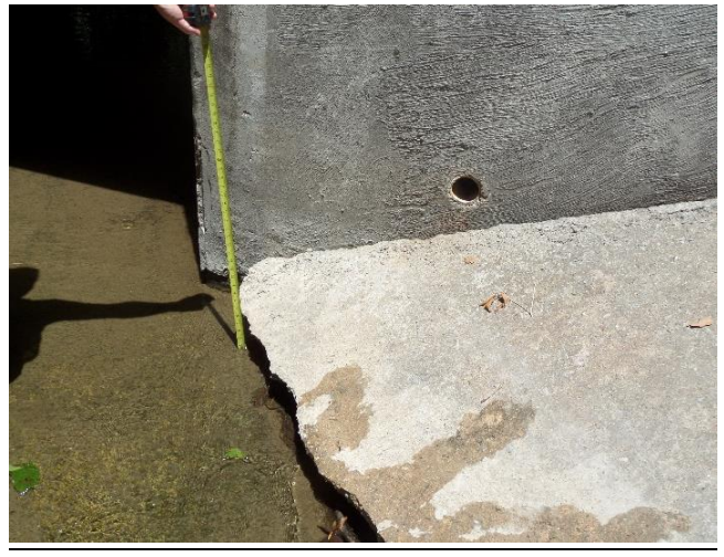
Toe exposed; chipping and undermining of riprap
