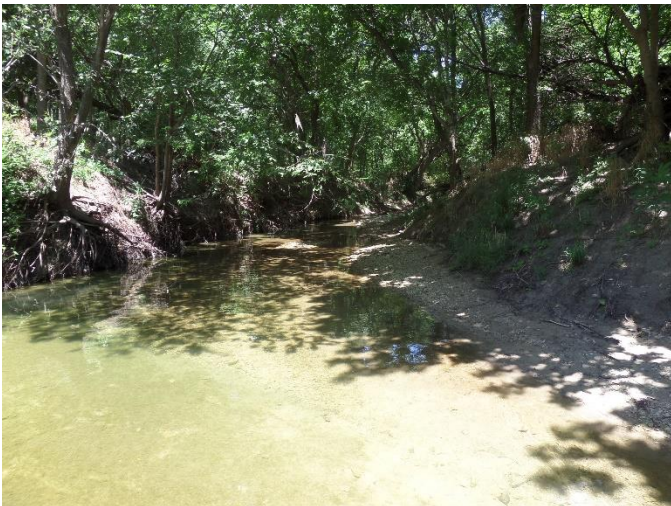
Moderate bank erosion looking upstream
