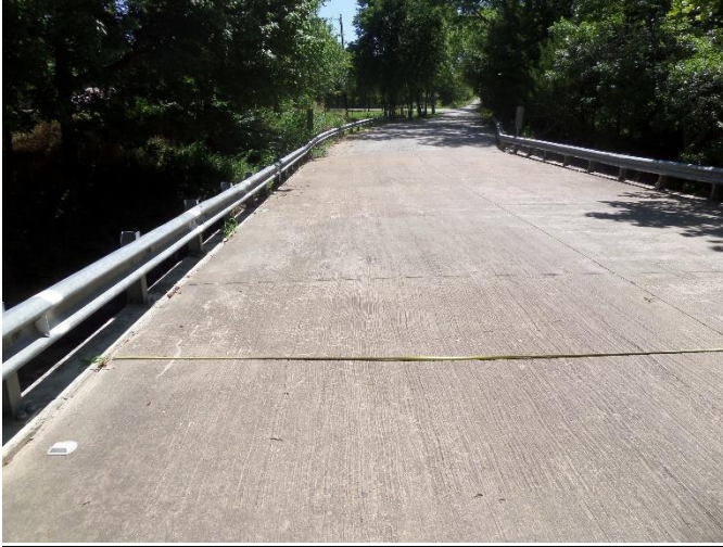
Lateral crack full width of roadway
