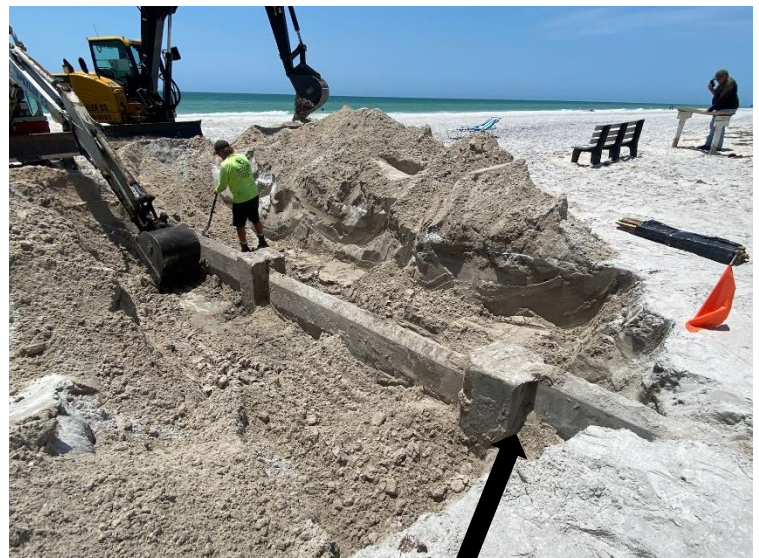
New Vinyl Sheets Set waiting for the concrete.
