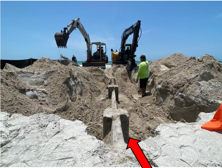
Original Beach Groins to be fortified with new vinyl sheets
