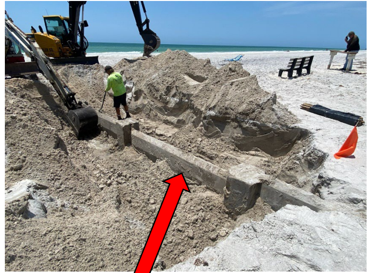
Original Beach Groins to be fortified with new vinyl sheets.
