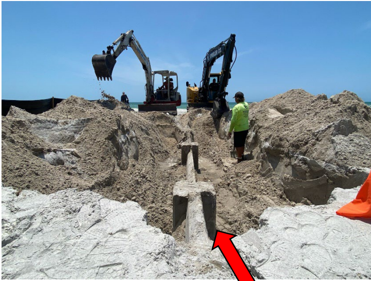
Original Beach Groins to be fortified with new vinyl sheets.
