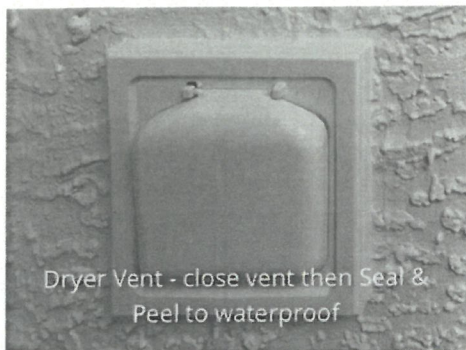
Dryer Vent - close vent then Seal & Peel to waterproof
