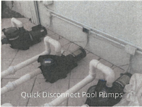
Plug and Play Pool Pump Electric (not hard wired)
