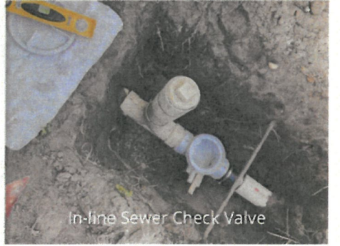
In-line Sewer Check Valve
