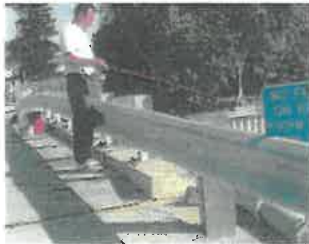
Existing Bridge Leading to Crystal Isles; Railing is Formed from Re-Used Highway Guard Rails
