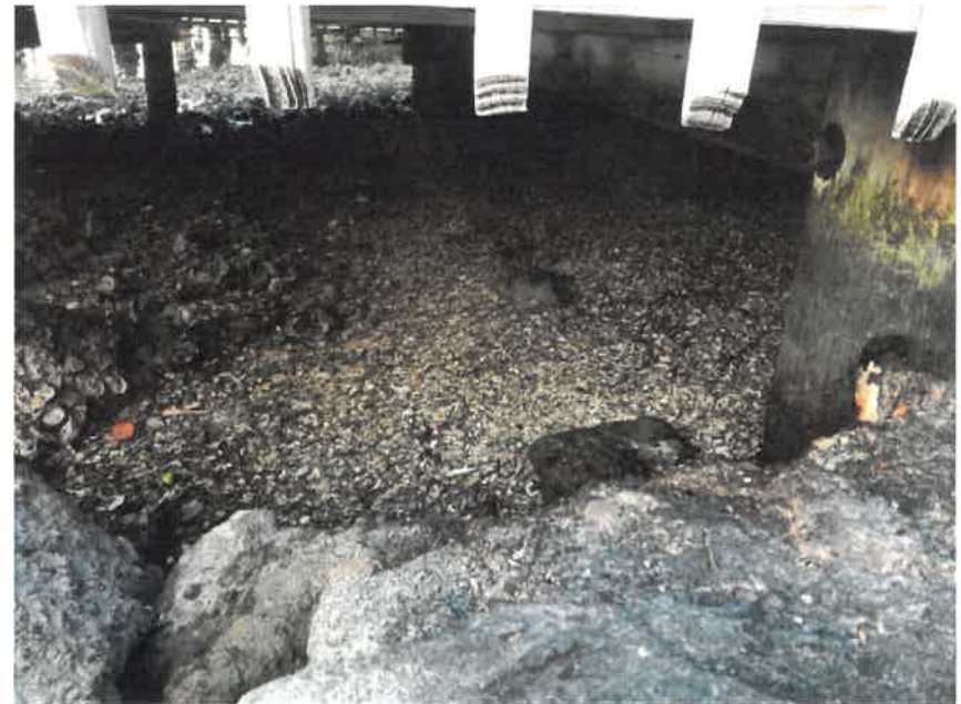
Poured concrete next door that retains/gathers sediment build-up making it shallow in the area
