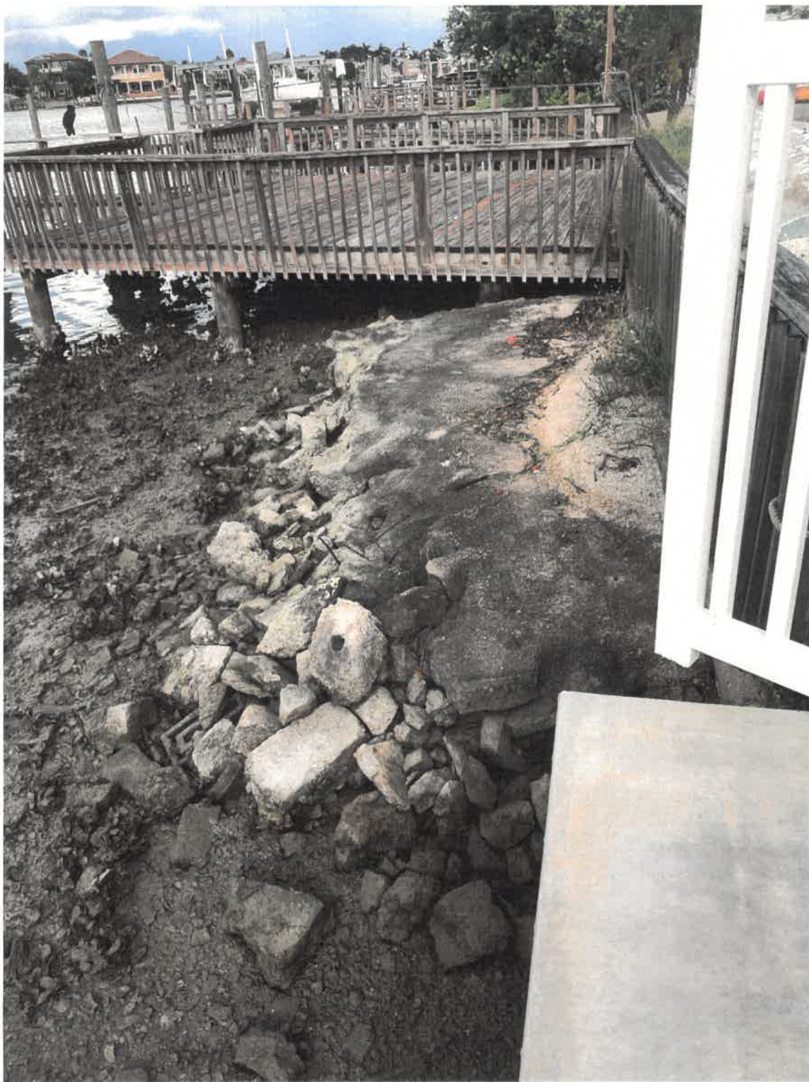
Poured concrete next door that retains/gathers sediment build-up making it shallow in the area
