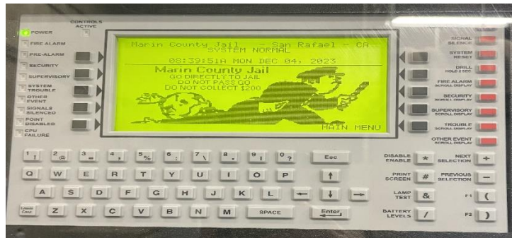
New Marin County Jail Fire Alarm Display Panel
