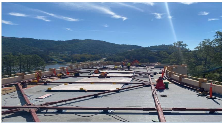
Placement and installation of new structural steel truss system on roof of Veterans Memorial Auditorium.
