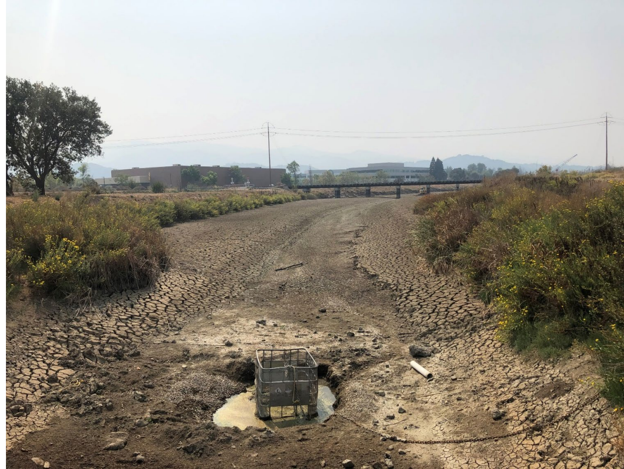
2020 Novato standard dredge – dewatered creek at downstream end
