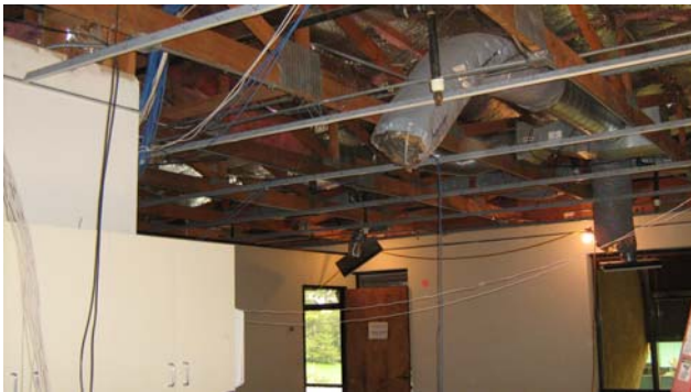
10 North San Pedro interior demolition
