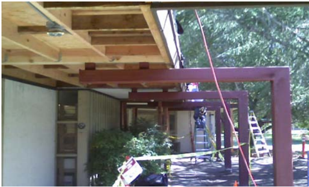
Juvenile Hall Re-roofing project
