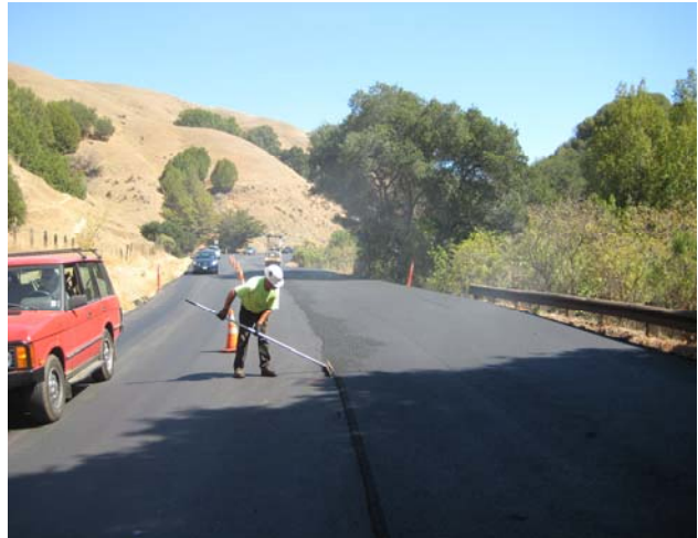
Repaving project along Sir Francis Drake Blvd.
