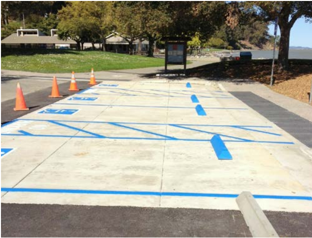
New accessible parking stalls at McNear's Beach
