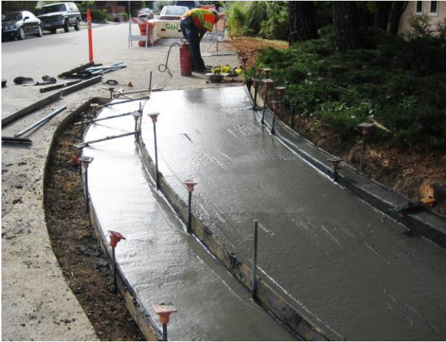
New accessible sidewalk and curb ramps
