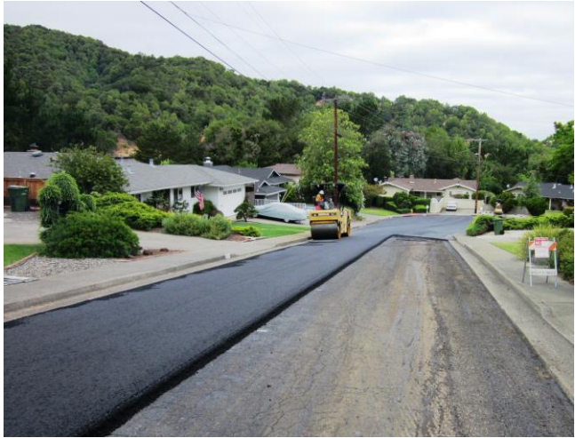
Residential – road re-paving
