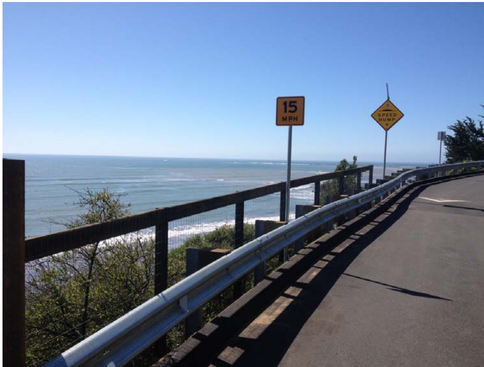
Terrace at Surfer's Overlook – Retaining Wall Repair
