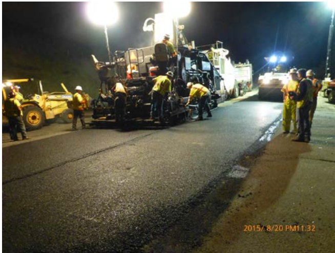
Road Rehabilitation Program – Southern Region
