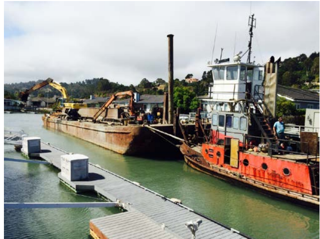
Dredger at Paradise Cay – CSA29 North Cay Channel B
