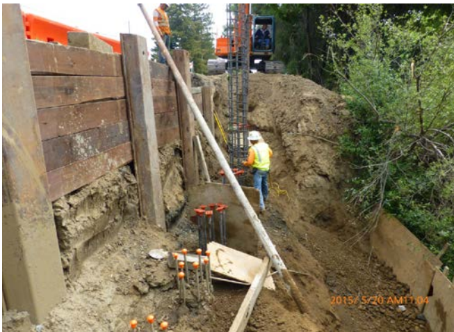
Emergency Slide Repair – Lucas Valley Road Milepost 1.66
