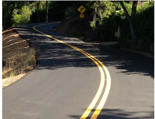
Road Rehabilitation Program – Central Region
