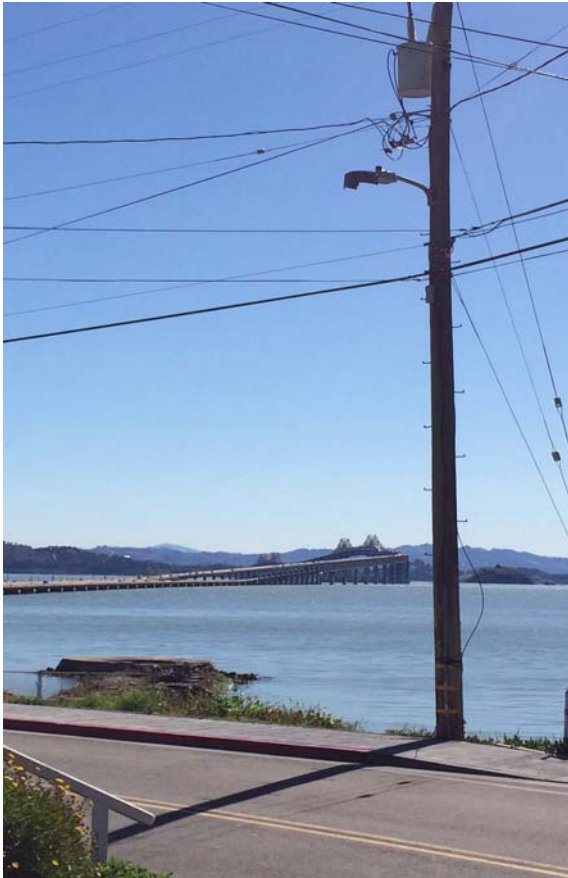
Power pole mounted light fixture
