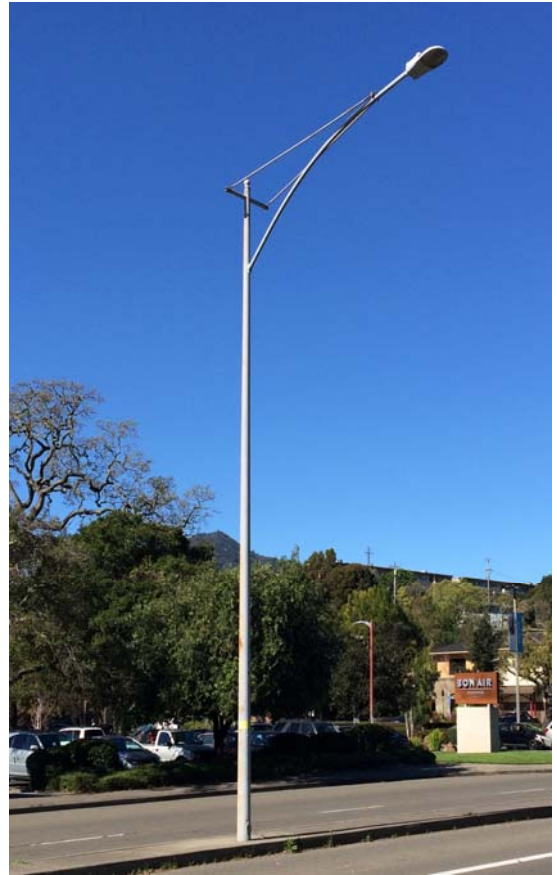
Steel light fixture pole
