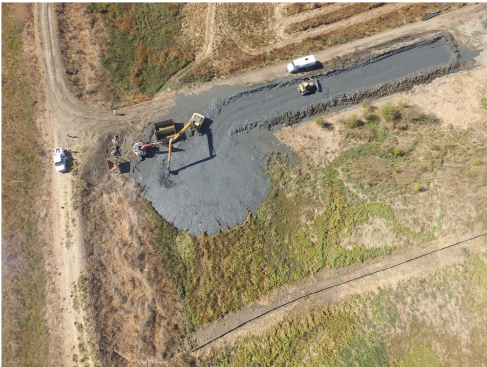
Aerial view of Ecotone Levee at Deer Island Basin during sediment placement
