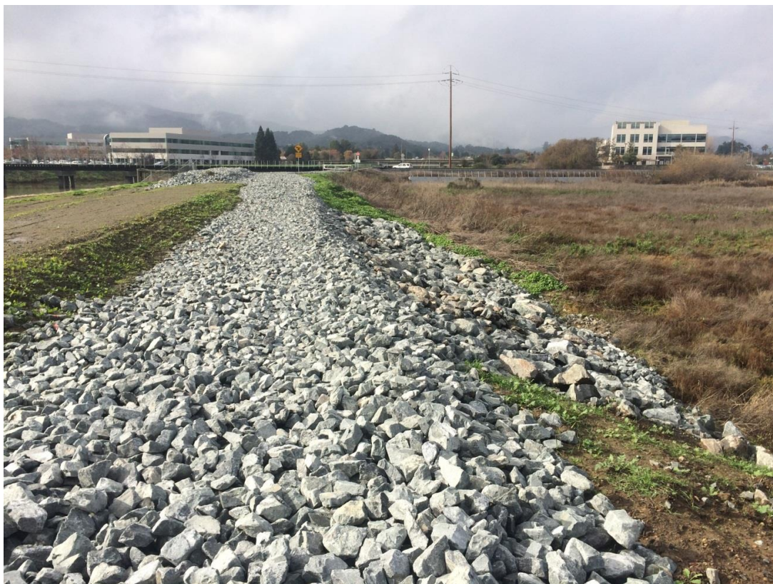
Completed Erodible Weir at Deer Island Basin/Novato Creek Levee
