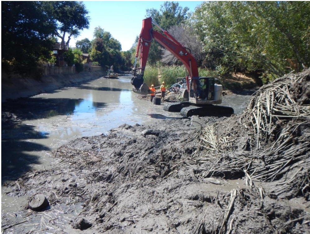
Excavators removing sediment and vegetative matter at Warner Creek
