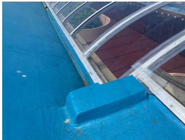
The project replaces skylights and skylight seals
