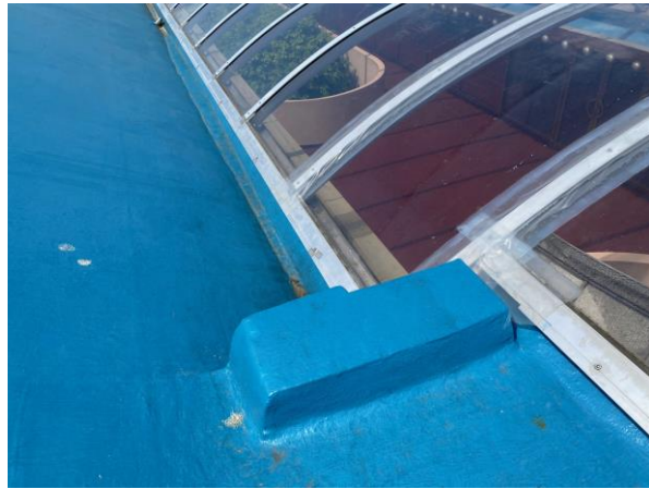
Third phase replaces skylights and skylight seals
