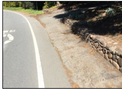
d) Narrow but rideable paved shoulder. Paving gravel parking area would create turnout.
