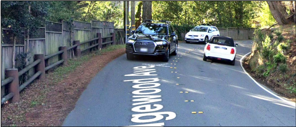
c) West curve, westbound approach (low metal barrier on south side)
