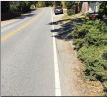
e) Unrideable gutter; encroaching landscape
