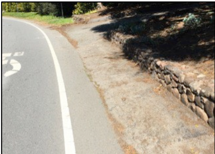
d) Narrow but rideable paved shoulder. Paving gravel parking area would create turnout.
