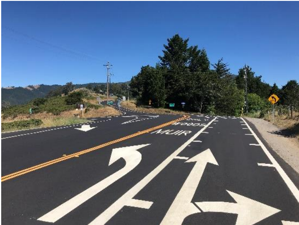
Northbound approach (Panoramic Highway)
