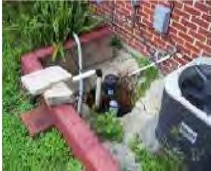
Figure 5.3: Sump Pump
