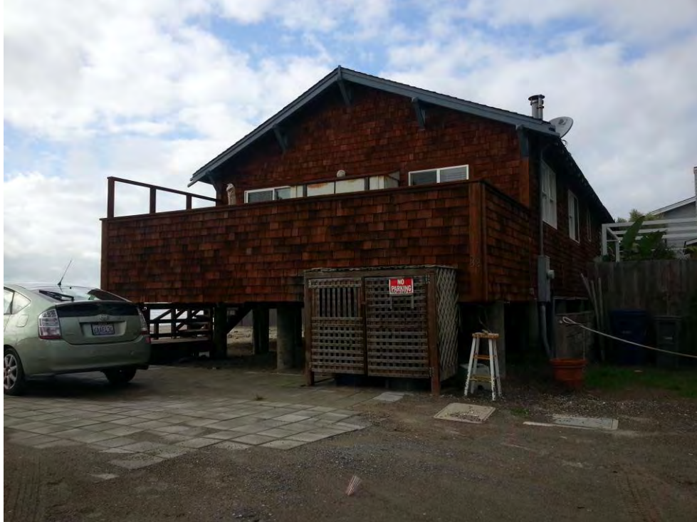
Figure 5.1 An Elevated House in the Study Area
