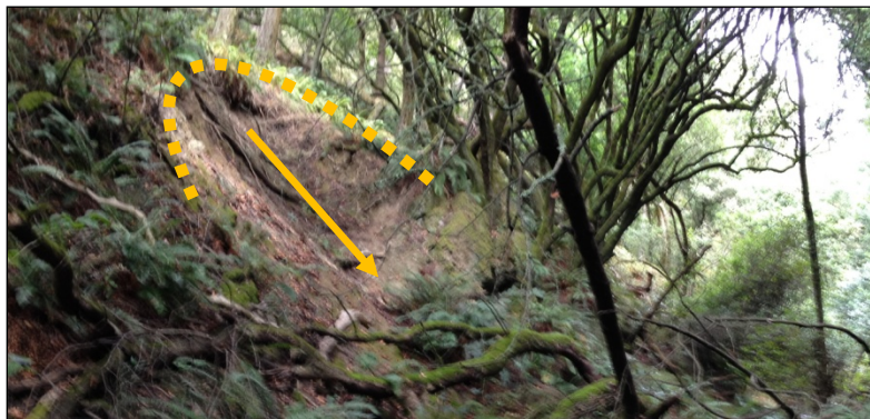
Figure 2-1 Recent debris slide scarp on an Easkoot Creek tributary near Table Rock.
