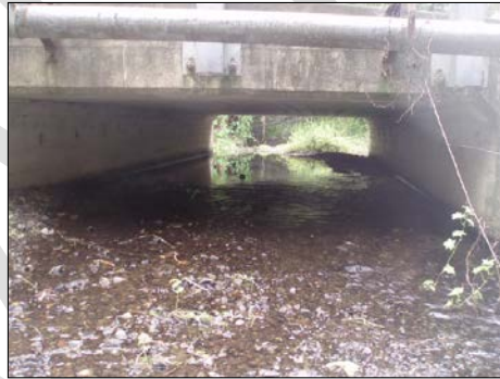
Figure ES6. Long-term sedimentation at Calle del Sierra can be seen by comparing conditions c. 1960 (left) and 2011 (right).
