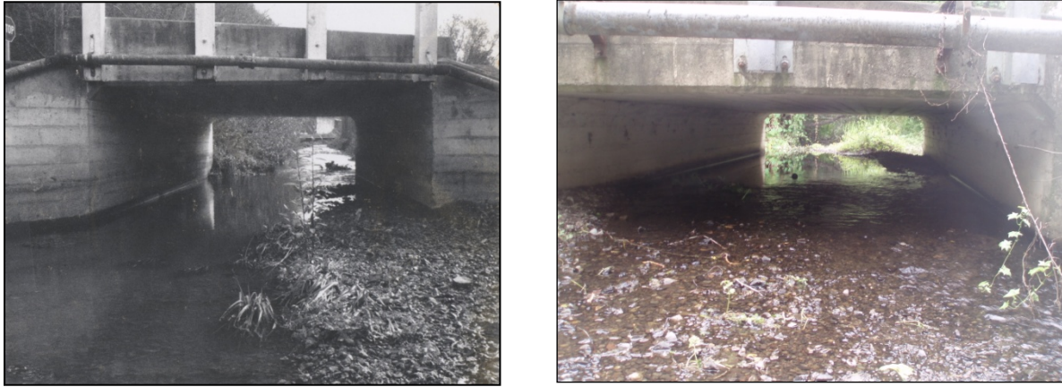
Figure 2-6 Long-term sedimentation at Calle del Sierra. Easkoot Creek c. 1960 (left) and 2011 (right).
