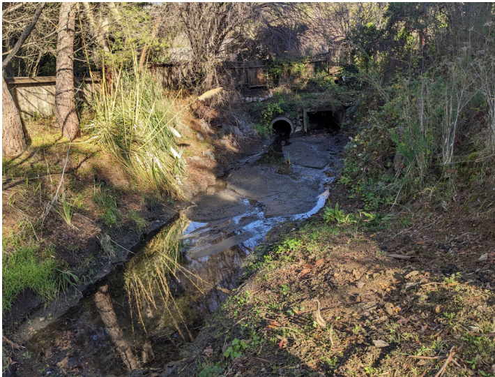
Photo 8. East Creek. Looking upstream to the outlet of culverts originating at or upstream from Karen Way (December 16, 2022). This is the maintained condition following channel maintenance dredging completed in October 2022. Note sedimentation near the culvert outfalls that occurred during November and December rainstorms.
