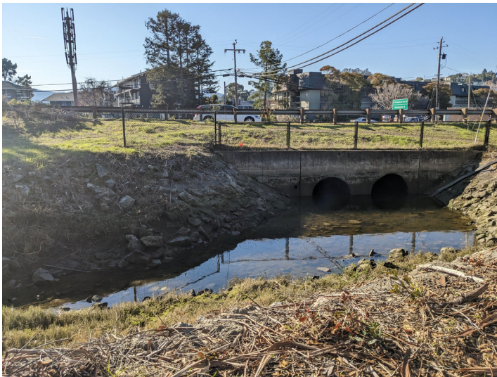
Photo 2. East Creek. Looking downstream from right bank of the grouted rock channel to the vertical concrete headwall inlet to the State Route 131 66" RCP "double-barrel" at Station 0+00' (December 16, 2022).
