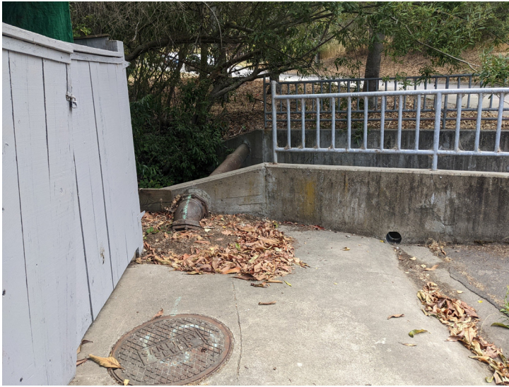
Photo 14. Upper East Creek. Looking from Cecilia Way to the upstream end of the right bank concrete transition channel wall about 30 feet upstream from the Cecilia Way culvert road crossing (August 17, 2022). The stormwater drain hole in the wall discharges creek flow onto the street during routine or average annual high creek flows. Blocking the drain hole combined with surface drainage improvements for directing the concrete swale flows to existing storm drain inlets near the Cecilia-Leland Way intersection should be considered.
