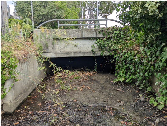
Photo 7. West Creek. Looking upstream to outlet of the Cecilia Way 5.3'x11.4' concrete box culvert (August 17, 2022). Note there is about 2-3 ft of fine sediment deposited within the downstream part of the culvert but much less sediment deposited in the upstream part of the culvert. This is the natural, unmaintained condition.
