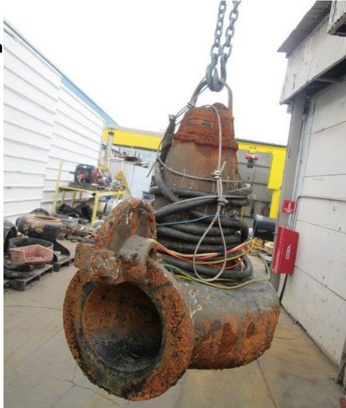
Seminary Drive Pump before 2025 refurbishment
