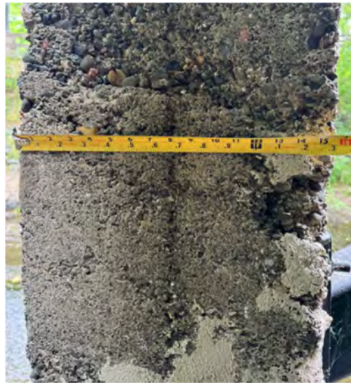
Example of Concrete Spalling Not Evaluated in Report
