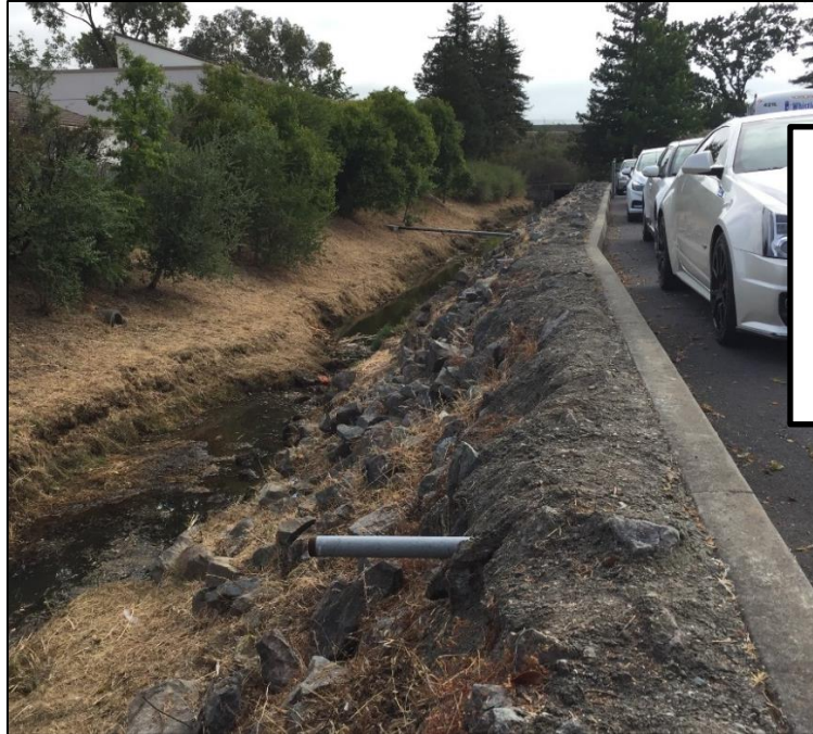
Merrydale Creek flood control and access easements looking towards Hwy 101
