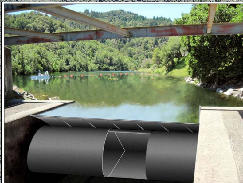
Conceptual view of the Phoenix Lake spillway with an inflatable/deflatable rubber dam raised by 6 feet, adding about 120 acre-feet of floodwater detention capacity.
