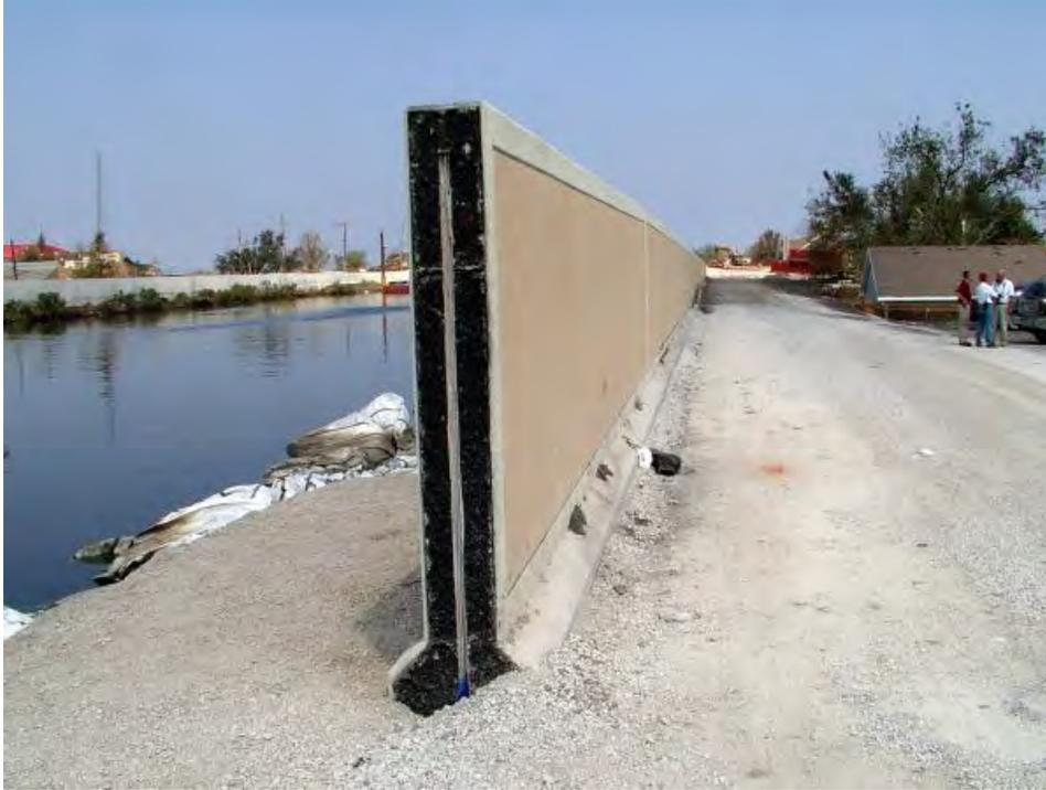
**Figure 3: Concrete Floodwall.**
