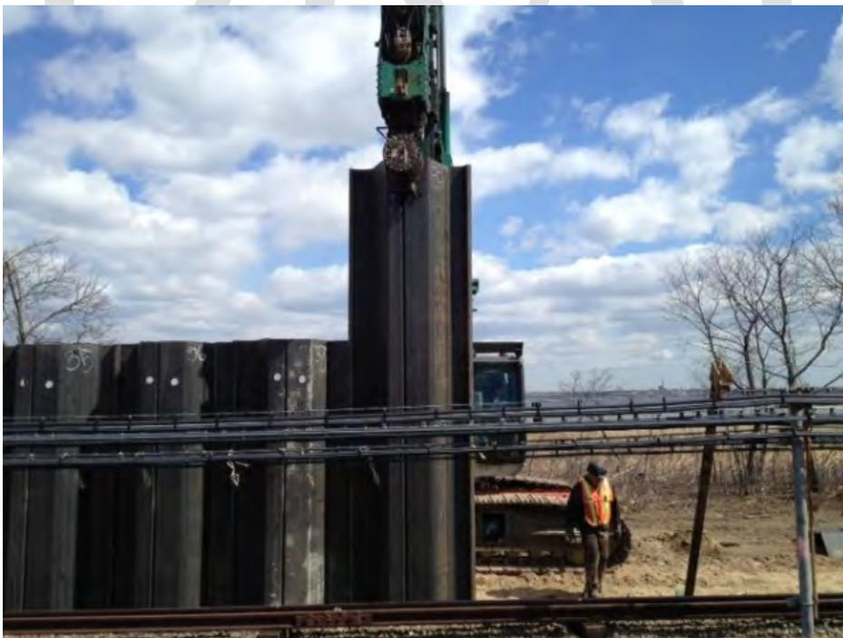
**Figure 4: Sheet Pile Wall.**
