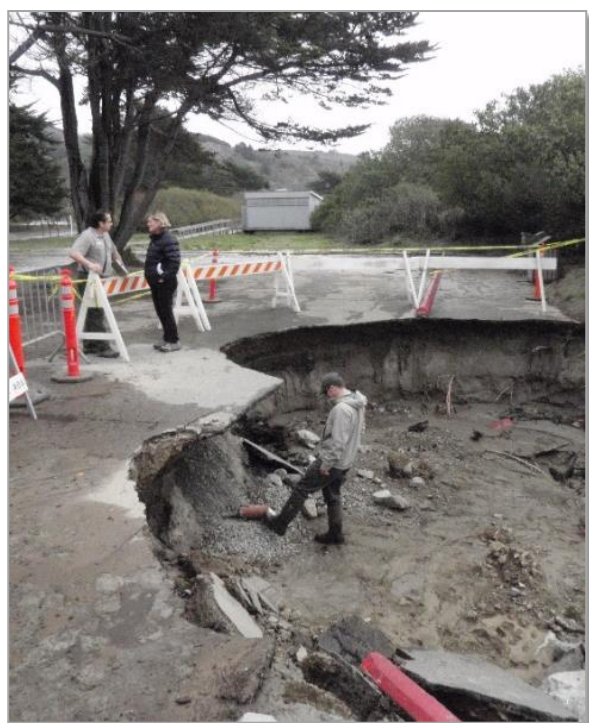
Figure 7.1: North Lot—Damage from Overtopping of Easkoot Creek
