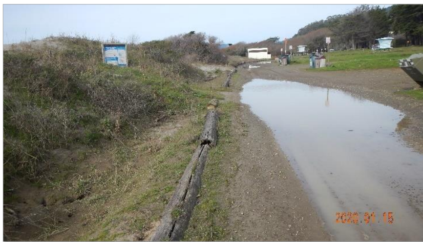
Figure 7.3: South Lot—Ponding Areas along the Dunes
