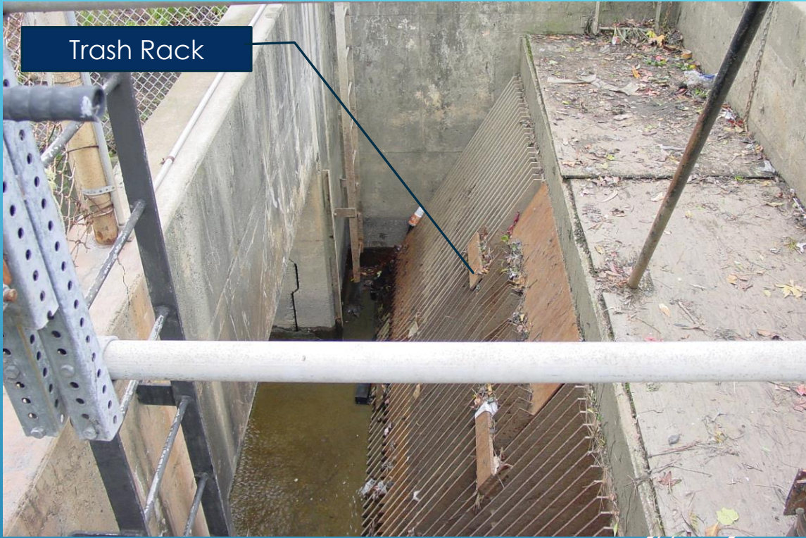
Kerner Blvd Pump Station
