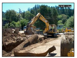
**After:** Replacement of the under-sized, pipe with an open-bottomed arched culvert opened up 1700' of habitat.
