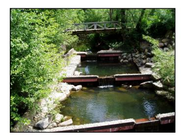
Barrier Removal Design: A fish ladder constructed in 1999 provides fish passage over a historic instream dam and includes a series of weirs large weir pools and a partial flow ladder for juvenile fish. Over time the Roy's Pools project has deteriorated and DFW has given the Golf Course a grant (2014) to redesign the structure including the County's bridge sill downstream.
