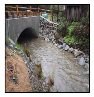
After: Replacement of the old pipes with an open-bottomed arched culvert allows salmonids to move freely up and down through the crossing, regardless of time of year and level of stream flows. Completion of the construction of this project removed the last major barrier to coho salmon in the Woodacre Creek watershed.
