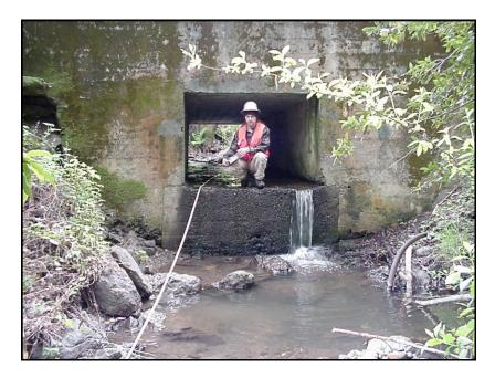
**After:** Replacement of the crossing with an open-bottomed arch allows the road crossing to literally become "invisible to the creek", providing passage for adult fish swimming upstream to spawn and juveniles migrating downstream during low flows in spring and summer.
