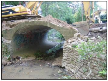
**After**: Restoration of this site included replacing the old culvert with an open bottomed arch, installing a roughened channel with embedded weirs to restore channel grade, and revegetating the adjacent stream banks with native plants from the watershed.
