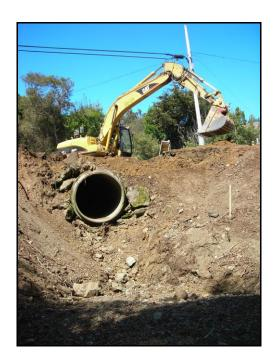
After: Replacement of the concrete pipe with an open-bottomed arched culvert allows the road crossing to become invisible to the creek; salmon can now pass under Muir Woods Road at all flows, with nothing to impede them.
