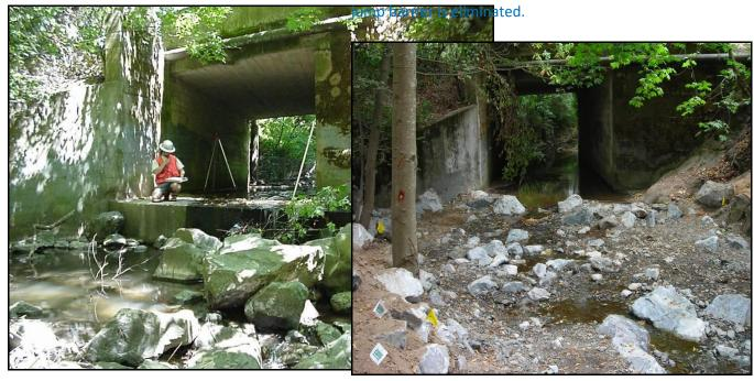
Salmon also faced a jump barrier getting into the box due to downstream scour caused by the increased velocities and were impeded by low flows in the summer when water sheeted across the concrete creating a low flow barrier to migration.
