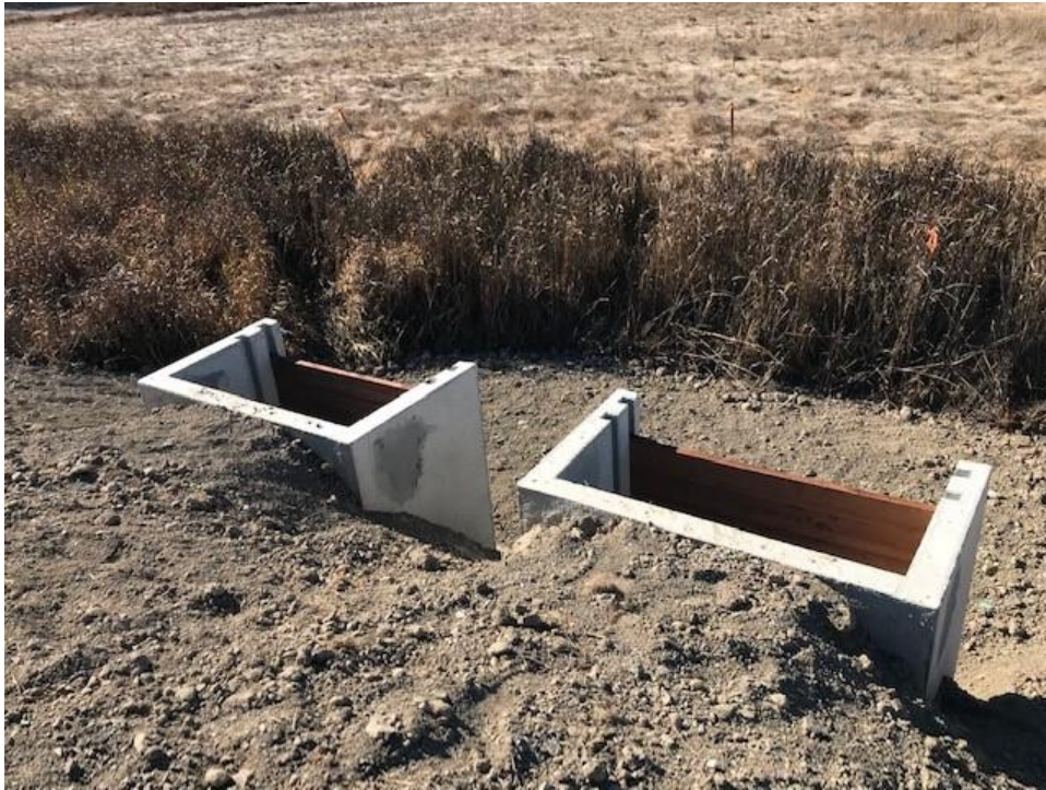
New water control structures to enhance seasonal wetlands at the Audubon property
