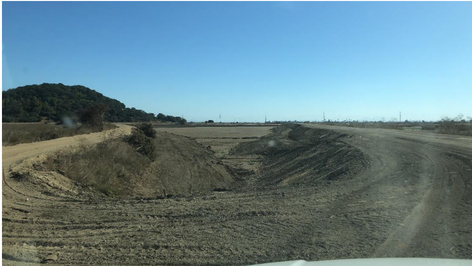
Heron's Beak pond in 2020 after placement of sediment removed from Novato Creek
