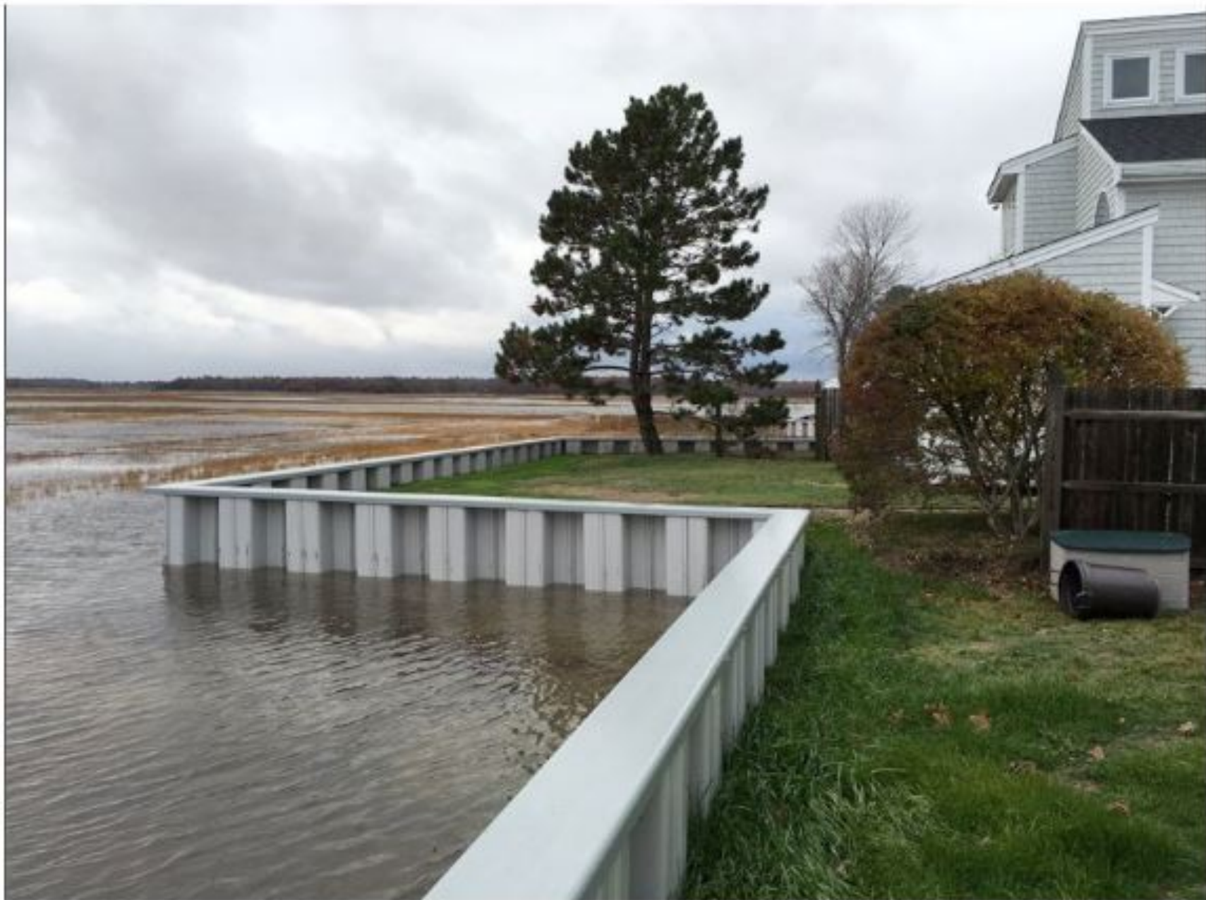
Figure 3-12: Sheet Pile Flood Wall
