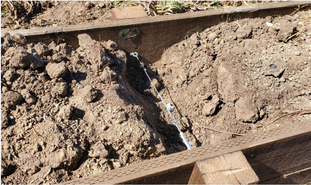
Figure 3-3: Steel Tieback
