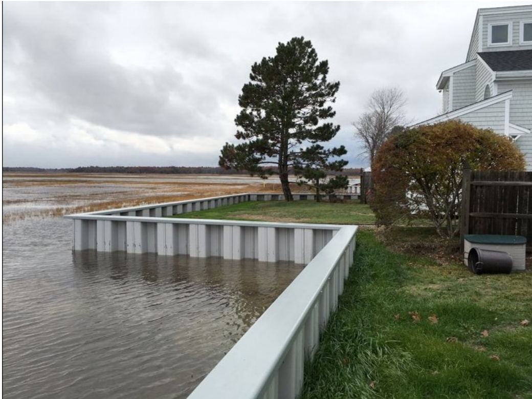
Figure 3-12: Sheet Pile Flood Wall
