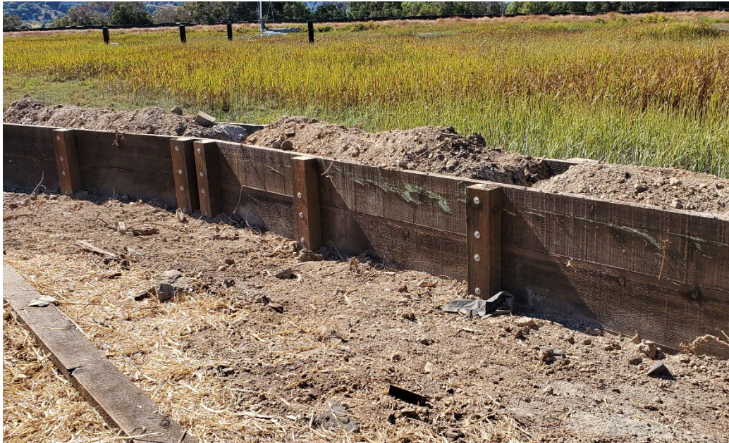
Figure 2-6: New TRB Section Under Construction
