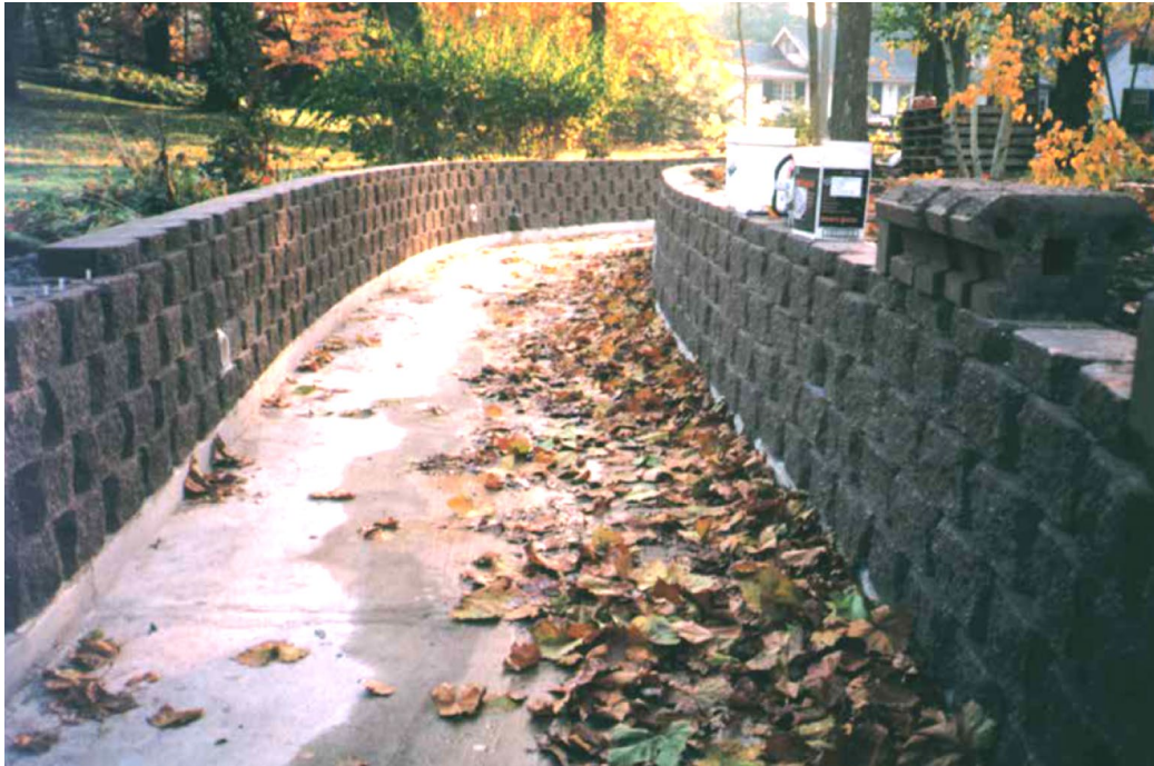
Figure 3-9: Creek Liner Using MSE Block Wall
