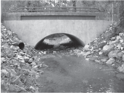
Arch culvert with natural stream bottom
