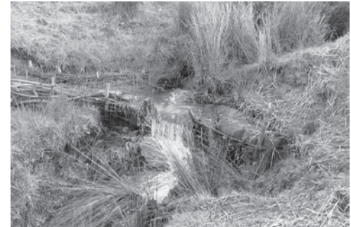
Willow wall headcut repair
