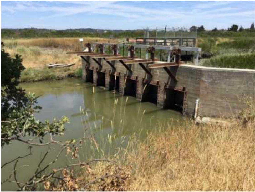
(a) Upstream Side
