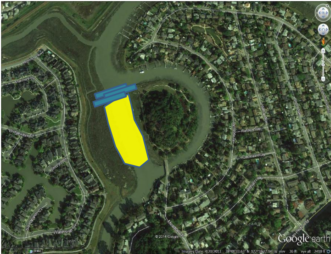
Figure 13: Concept for a low-flow blockage of outer channel at Santa Margarita Island, with wetlands forming upstream
