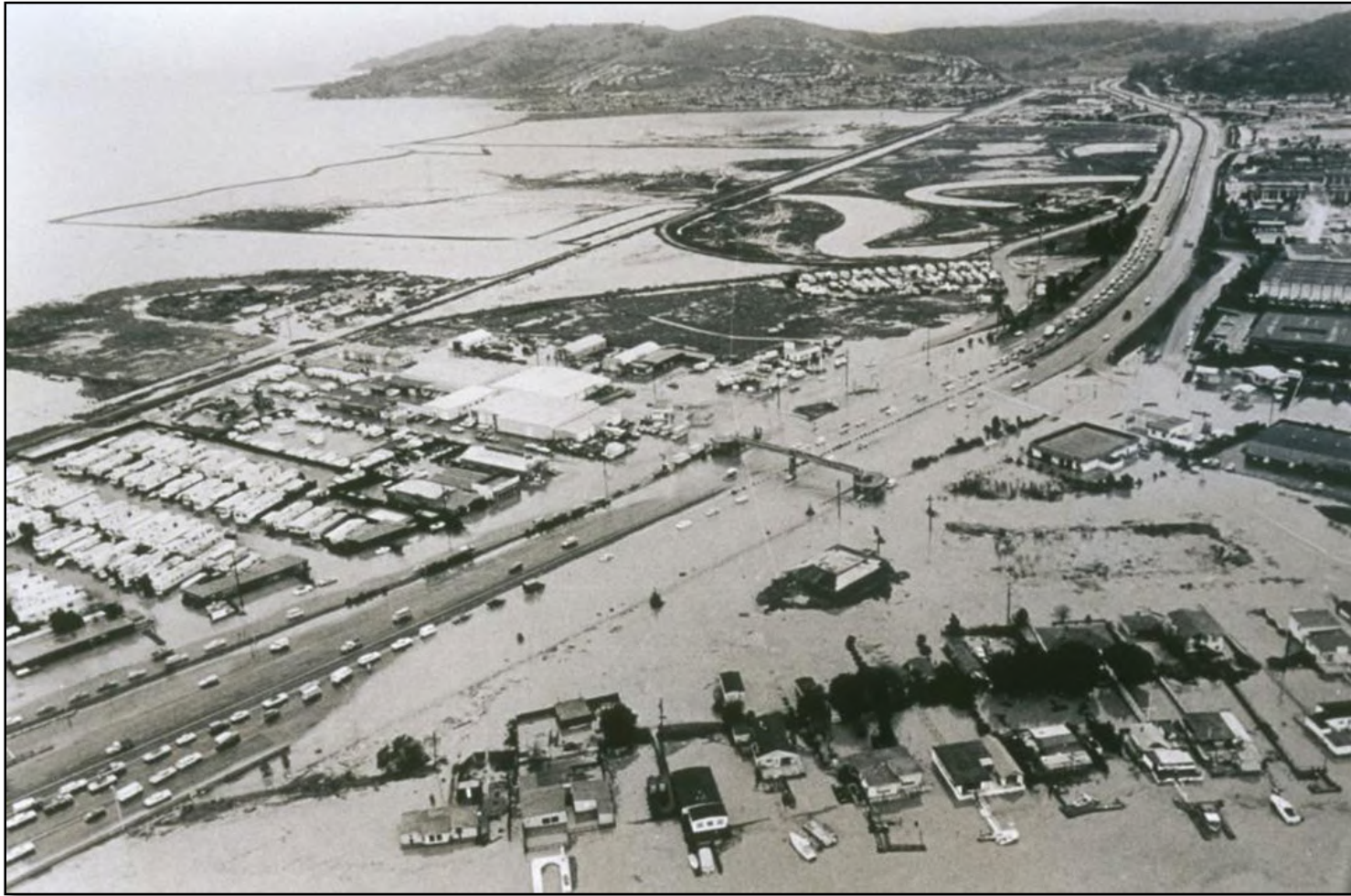
1973, Larkspur & Corte Madera (Hwy 101) High Tide and Storm Flooding Event
