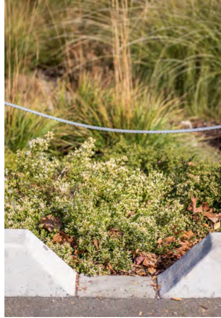
Drainage & Stormwater Treatment
