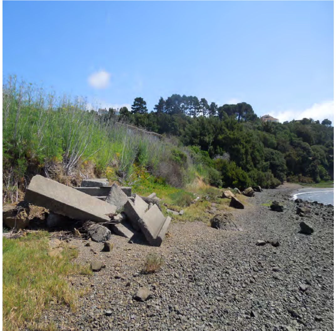
Eroded Seminary Drive shoreline east of the rock slope protection, with collapsed access structures. June 21, 2012
