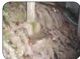
Visible erosion under a deck is common.
