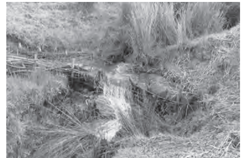
Willow wall headcut repair
