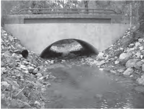
Arch culvert with natural stream bottom
