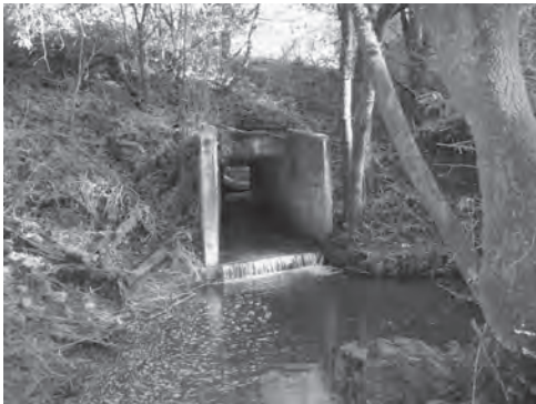
Traditional box culvert with concrete bottom
