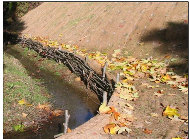
Biotechnical bank stabilization using gently-sloped banks and a small, inset floodplain protected with a willow wall. The floodplain and bank were later planted with native plants. Photo by Prunuske Chatham, Inc.
